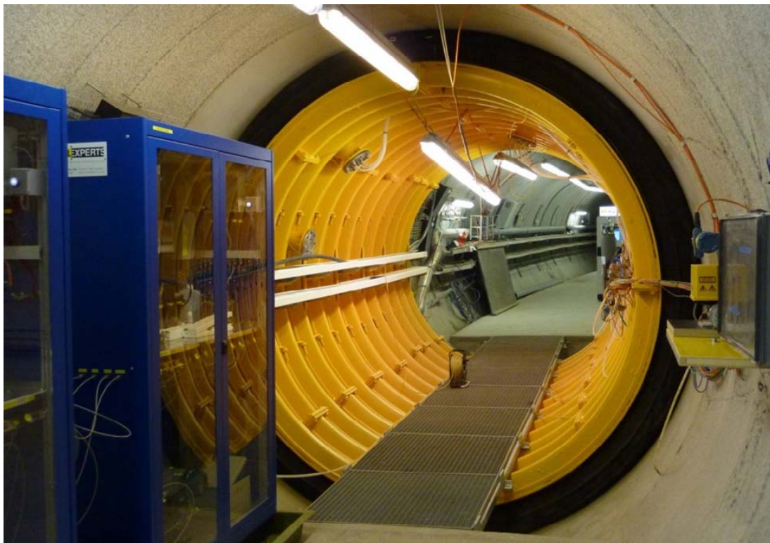
Figure 3-32. CFM field test bed at Grimsel Test Site: Tunnel packer system used to isolate the shear zone (from http://www.grimsel.com/gts-phase-vi/cfm-section/cfm-site-preparation ). Small disks with tubing issuing from them (inside yellow packer) are “surface packers” that seal the tunnel wall and collect water from inflow points. Tunnel diameter is 3.5 meters.
