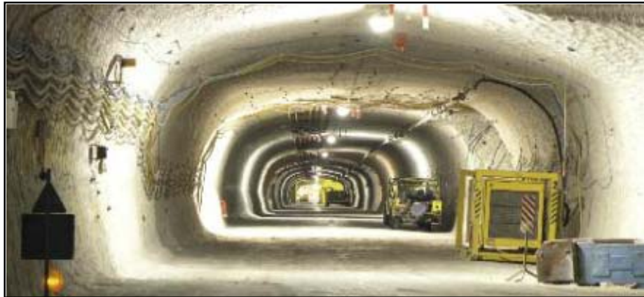
Figure 4-5. View of one of the underground tunnels at Gorleben site at the 840 m level (from BMWi, 2008)
