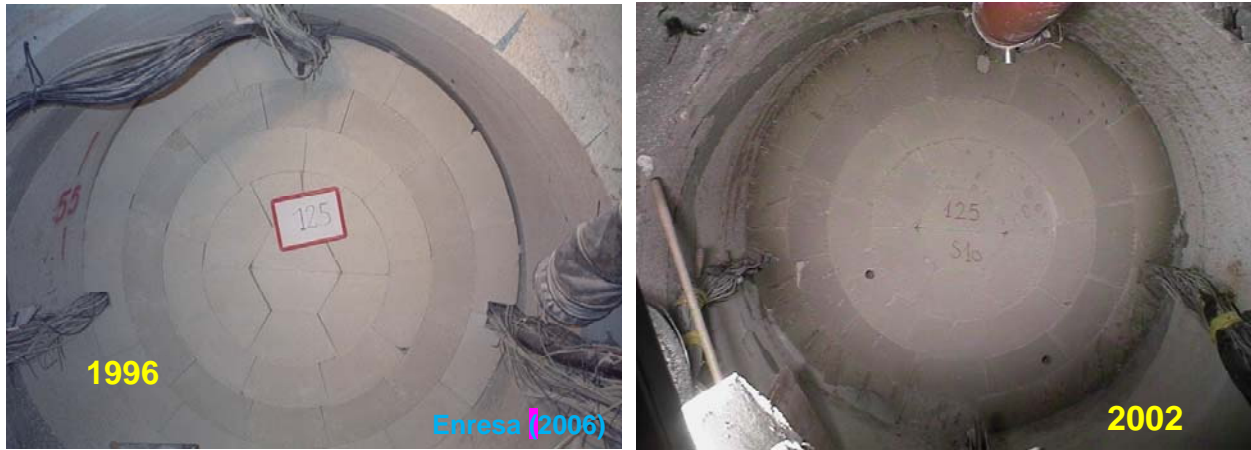
Figure 3-36. Bentonite blocks during installation of the experiment in 1996 (left) and after the first dismantling in 2002 (right). In 2002, all initial emplacement gaps between blocks were closed. (from NAGRA, 2014)
