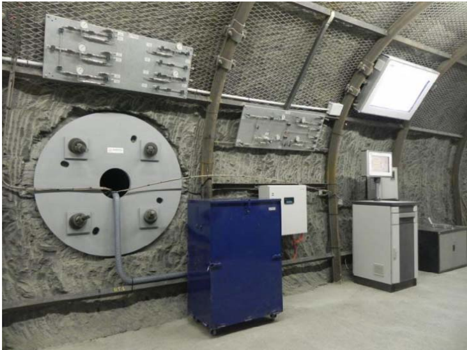
Figure 3-3. SEALEX Experiment at the Tournemire URL: View of mini-tunnel from gallery after seal emplacement (from Barnichon, 2011)
