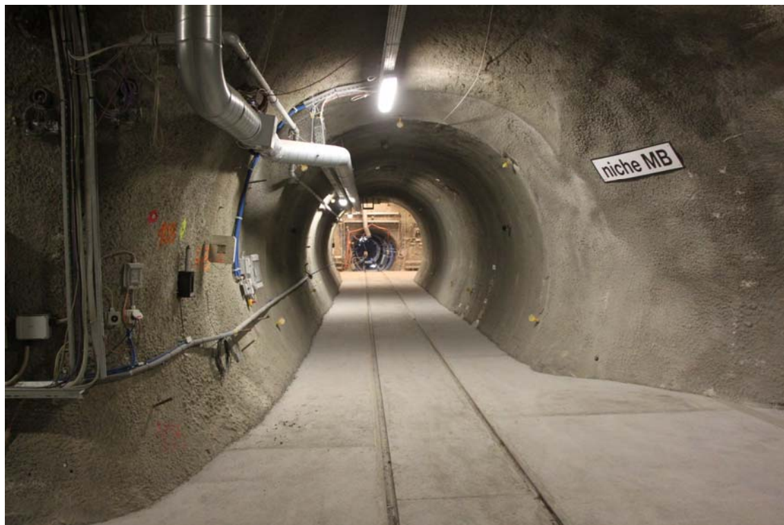
Figure 3-24. View from the FE gallery into the heater tunnel during final installation (from Bossart, 2014a)
