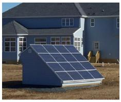
Tindall Homes installed their optional grid-tied solar photovoltaic systems on backyard garden sheds, situated for maximum solar gain. Wiring for the systems runs underground from the shed to the home's basement.
