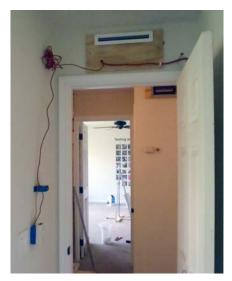
Through-wall fans move conditioned air from the hallway into the bedrooms of the Pittsburgh new construction unoccupied test house.
