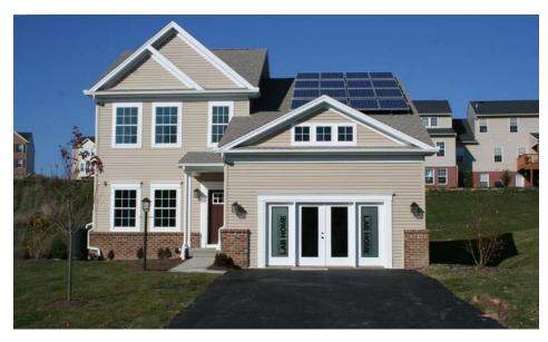
The new construction two-story unoccupied test house faces south, has poorly shaded windows, and includes basement construction.
