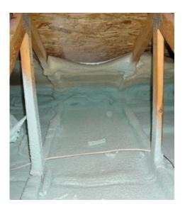
Spray foam is used to insulate and air seal the attic floor and any ducts located in the attic. The spray foam is covered with more than 12 inches of blown cellulose for the equivalent of R-49 of attic insulation.
