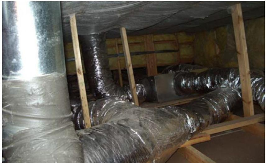
The builder worked with Building Science Corporation to design an insulated attic to provide a protected environment for the home's air source heat pump and ducts.
