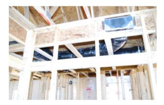
Artistic increased the efficiency of its heating and cooling systems by putting ducts in conditioned space in a central chaise down the main hallway.
