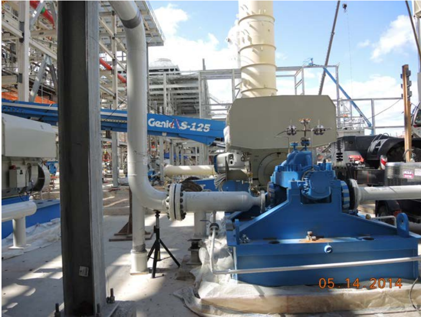
Train 1 installing pipe on solvent charge pumps
