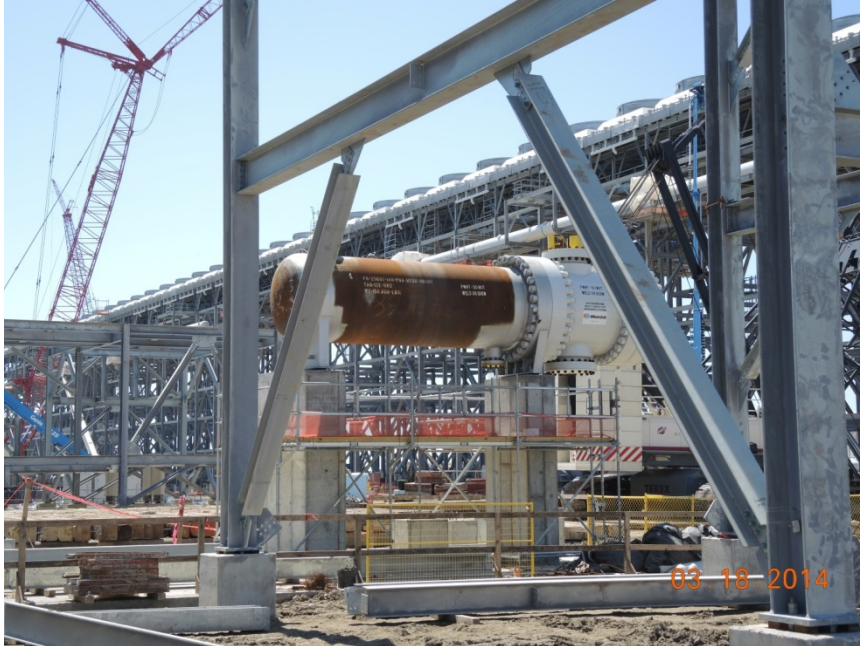
Train 2 installed feed gas heater.
