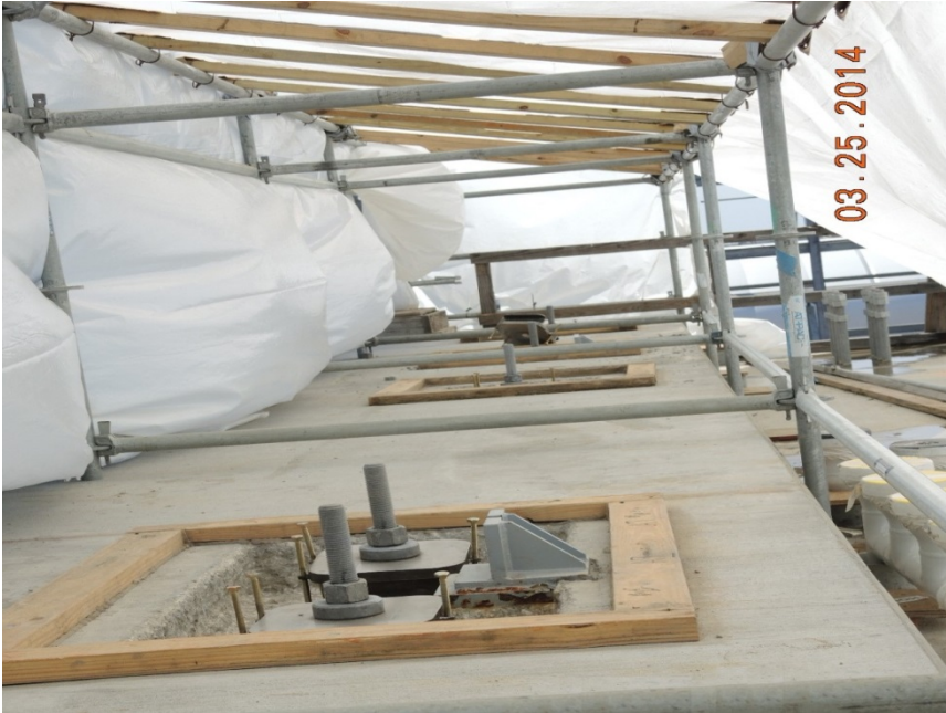
Train 1 ethylene turbine & compressor sole plates.
