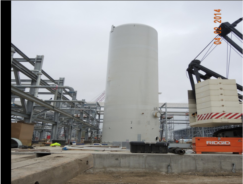
OSBL installation of instrument air receiver
