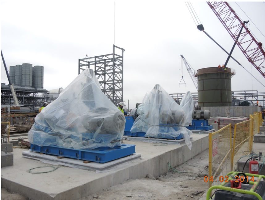
Train 2 setting of lean solvent booster pumps
