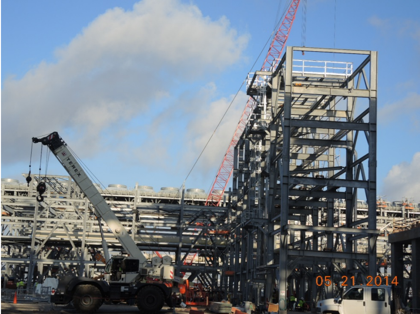
Train 2 steel installation
