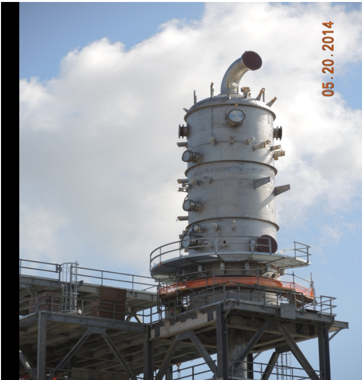
Train 1 installing platforms on heavies removal column
