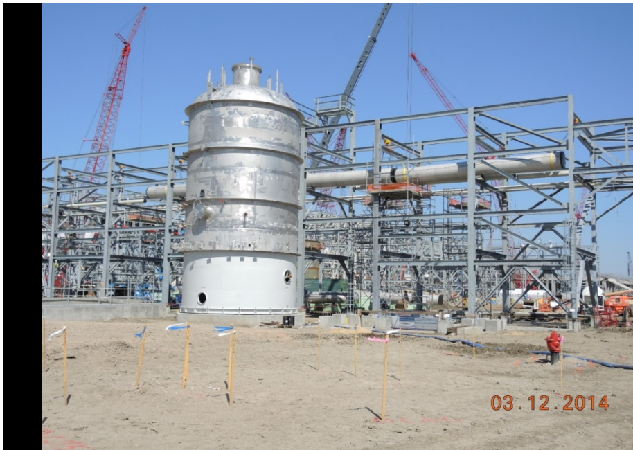
OSBL installing pipe to BOG Recycle KO Drum.
