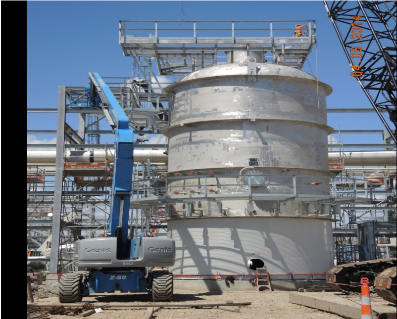
OSBL installing platforms on BOG recycle KO drum
