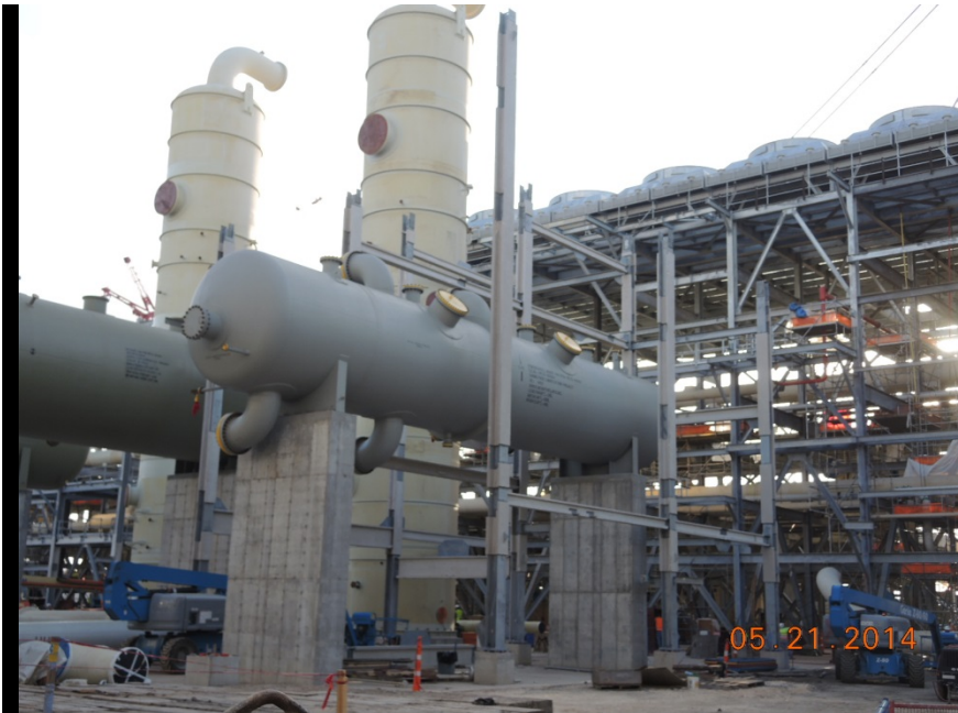
Train 1 installing steel around HS propane methane ethylene chiller
