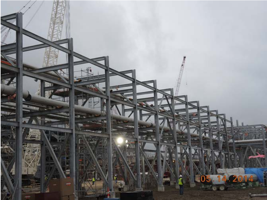
OSBL installing pipe
