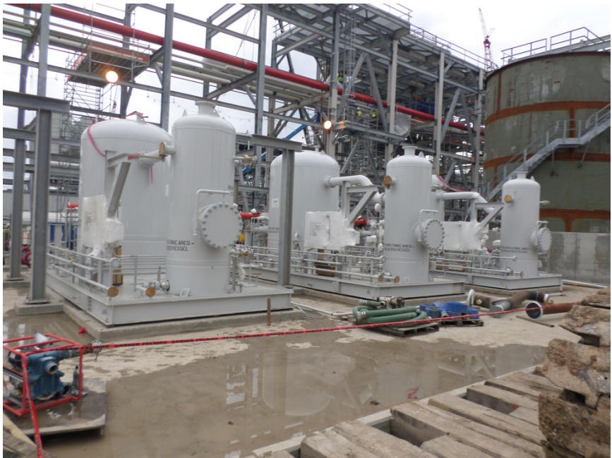
Train 1 H2S removal package skids installed
