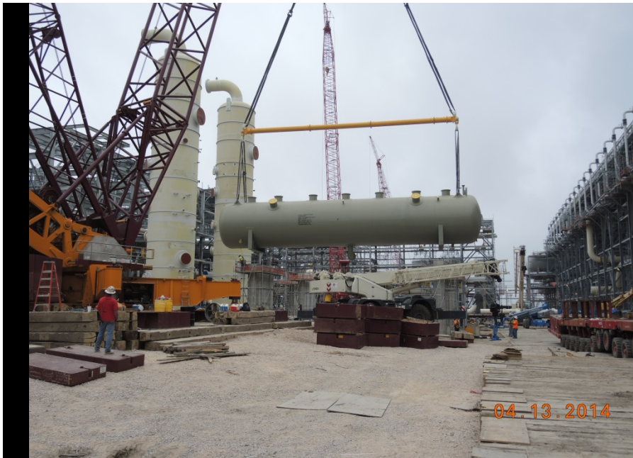
Train 1 setting LS propane-ethylene cond/feed chiller
