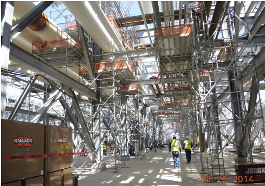
Train 1 scaffolding and pipe installation.
