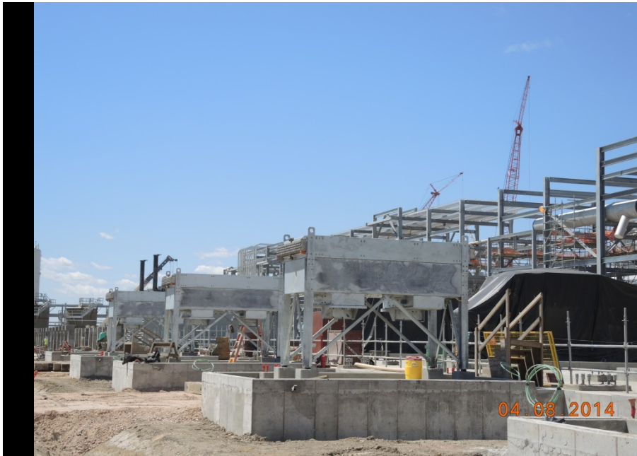
OSBL setting BOG compressors and BOG compressor lube oil coolers
