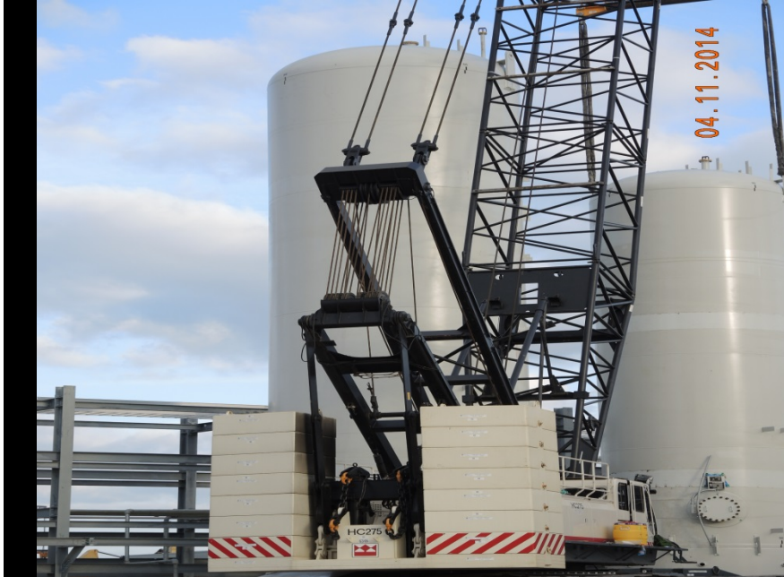
OSBL setting nitrogen receiver tank
