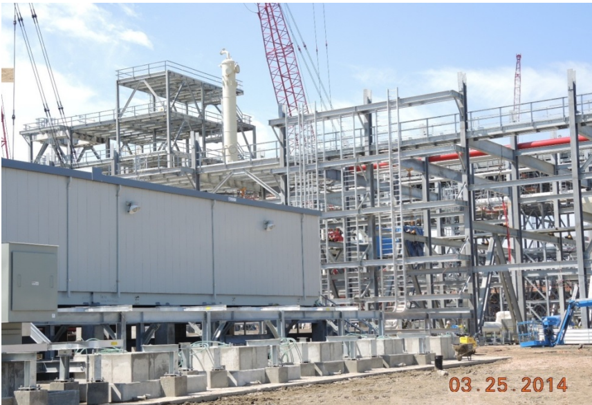
Train 1 installing cable tray to Compressor Substation.
