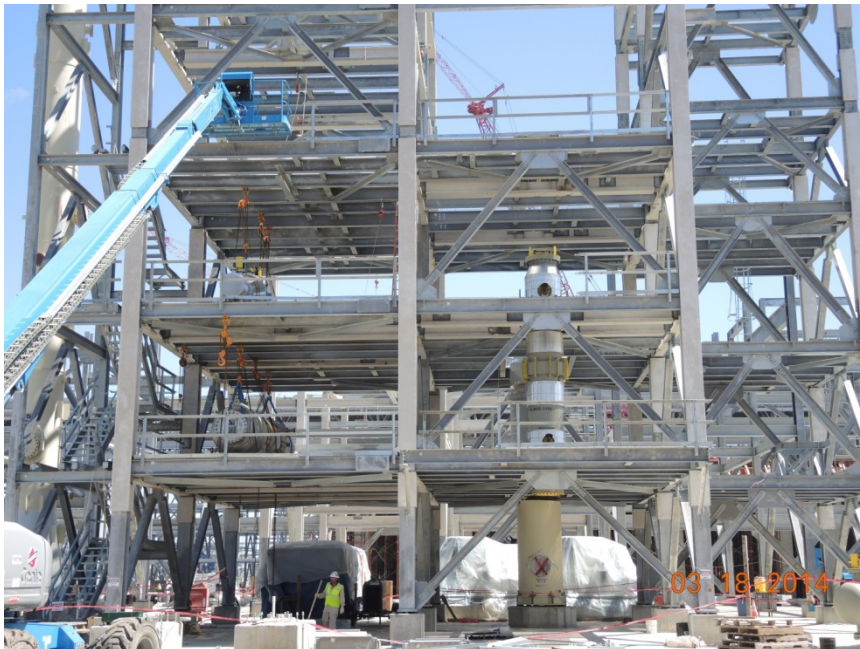
Train 2 setting equipment.
