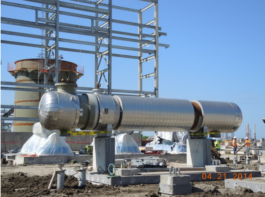
Train 2 setting regenerator reboiler
