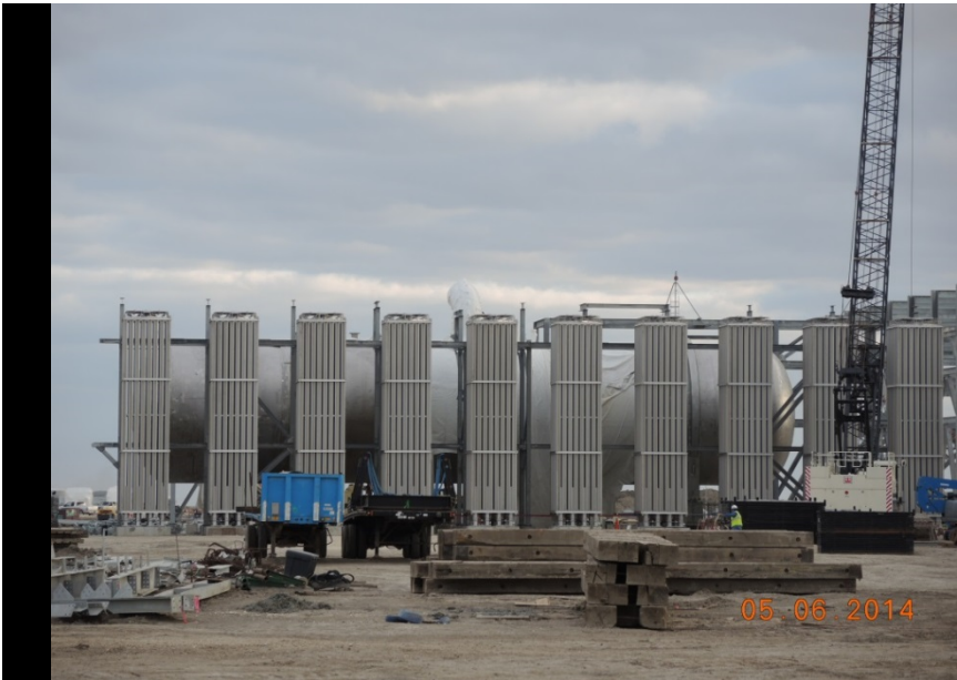
OSBL setting dry gas flare vaporizer
