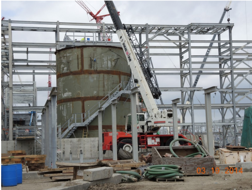
Train 1 installing stairs and platform on water tank.
