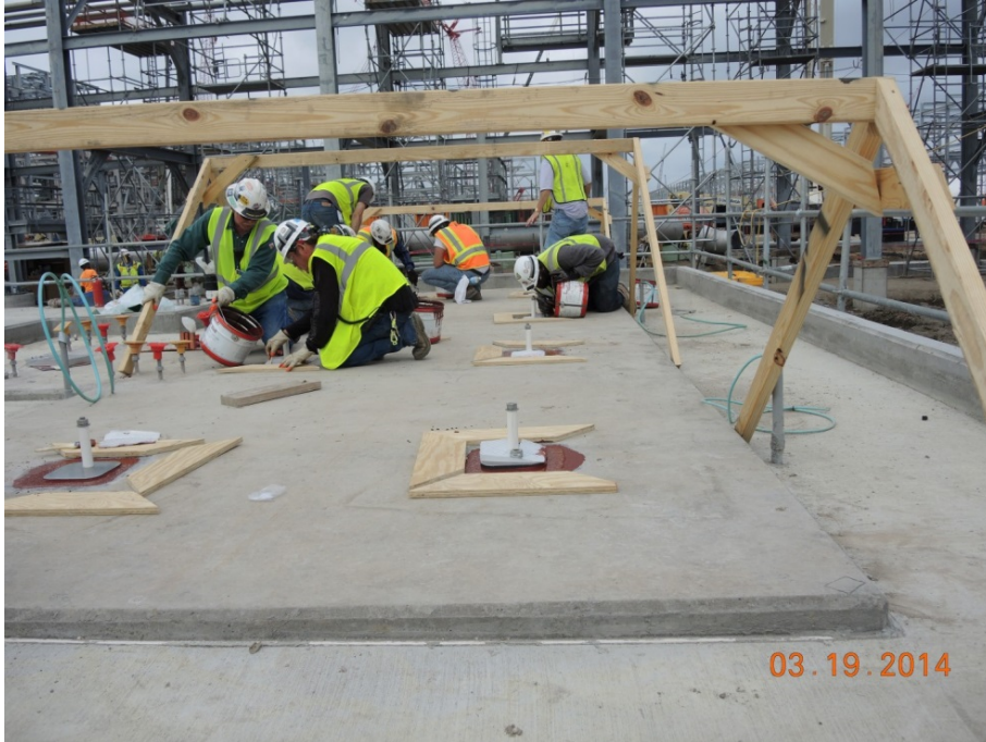
OSBL grouting BOG compressors sole plates.
