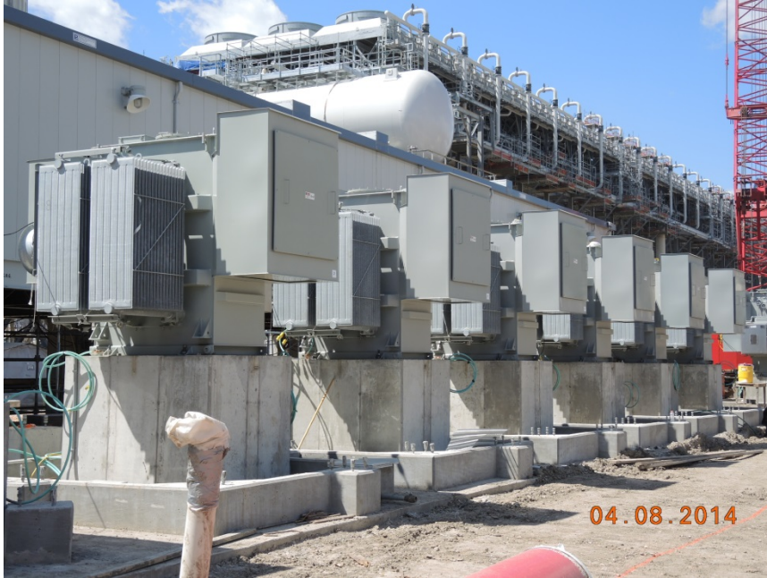
Train 1 setting propane substation transformers
