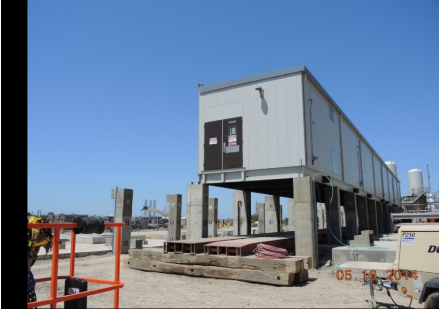
OSBL setting utility substation
