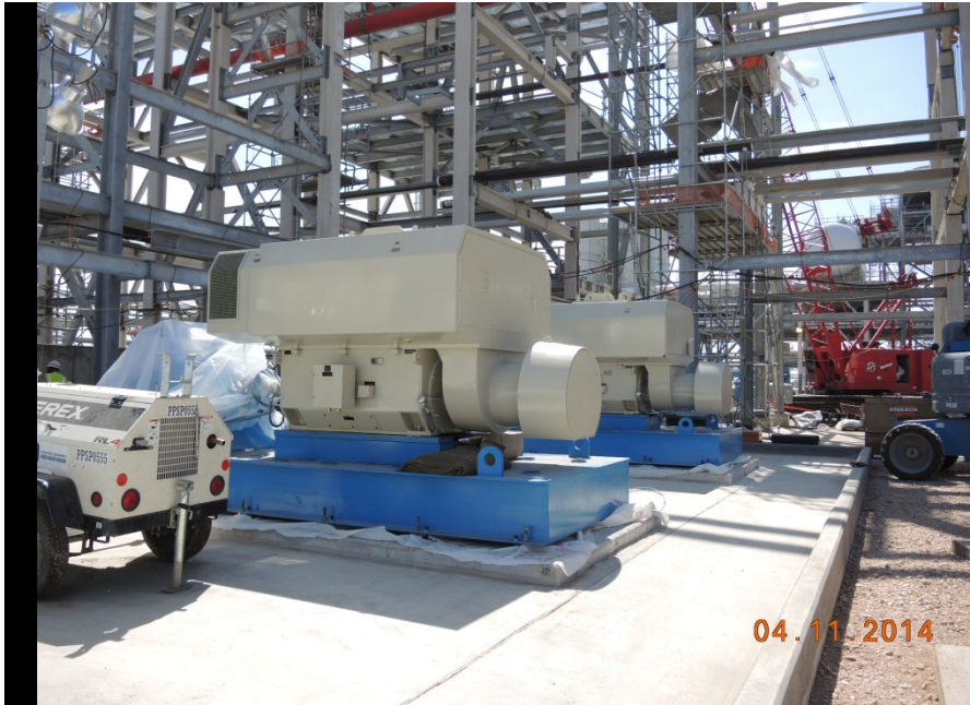
Train 1 lean solvent charge pumps set in place
