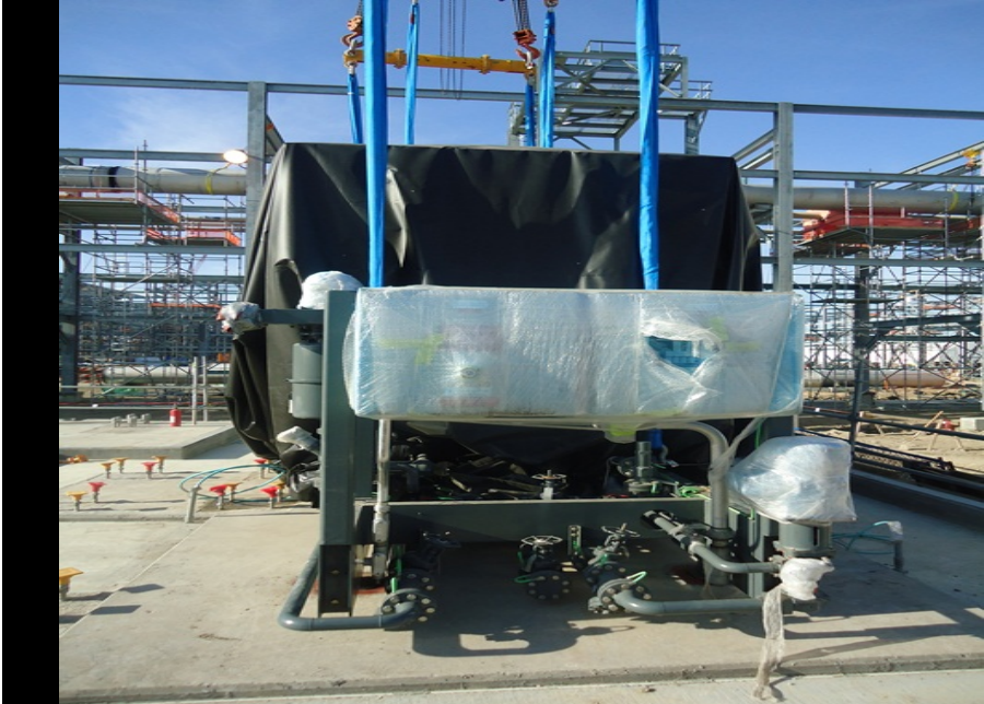
OSBL setting of BOG compressor
