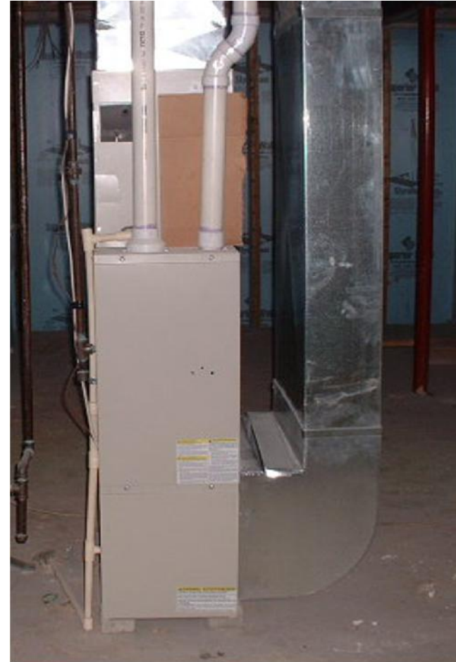
Direct-Vent Furnace
