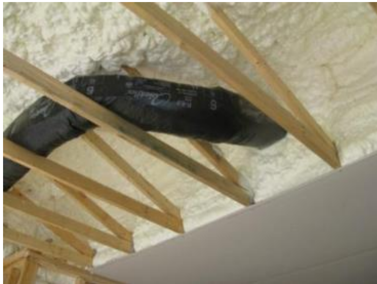
Ducts in unvented attic
