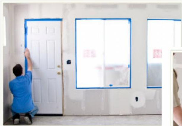
Engineer Curtis Harrington taping off areas in preparation for sealing.
