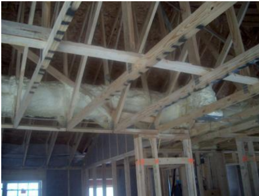
Option 1- prior to ceiling gypsum board
