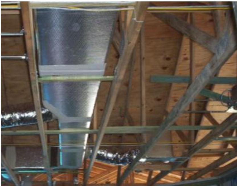
Option 1- prior to ceiling gypsum board
