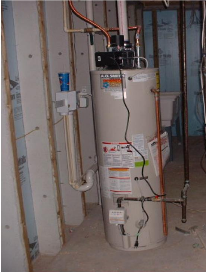
Power Vented Water Heater
