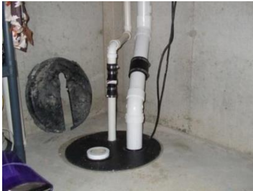
Sealed Sump Pump
