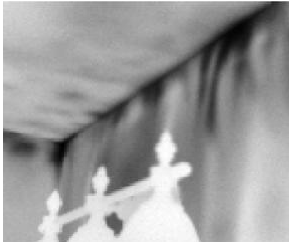
Attic air infiltration into the wall
