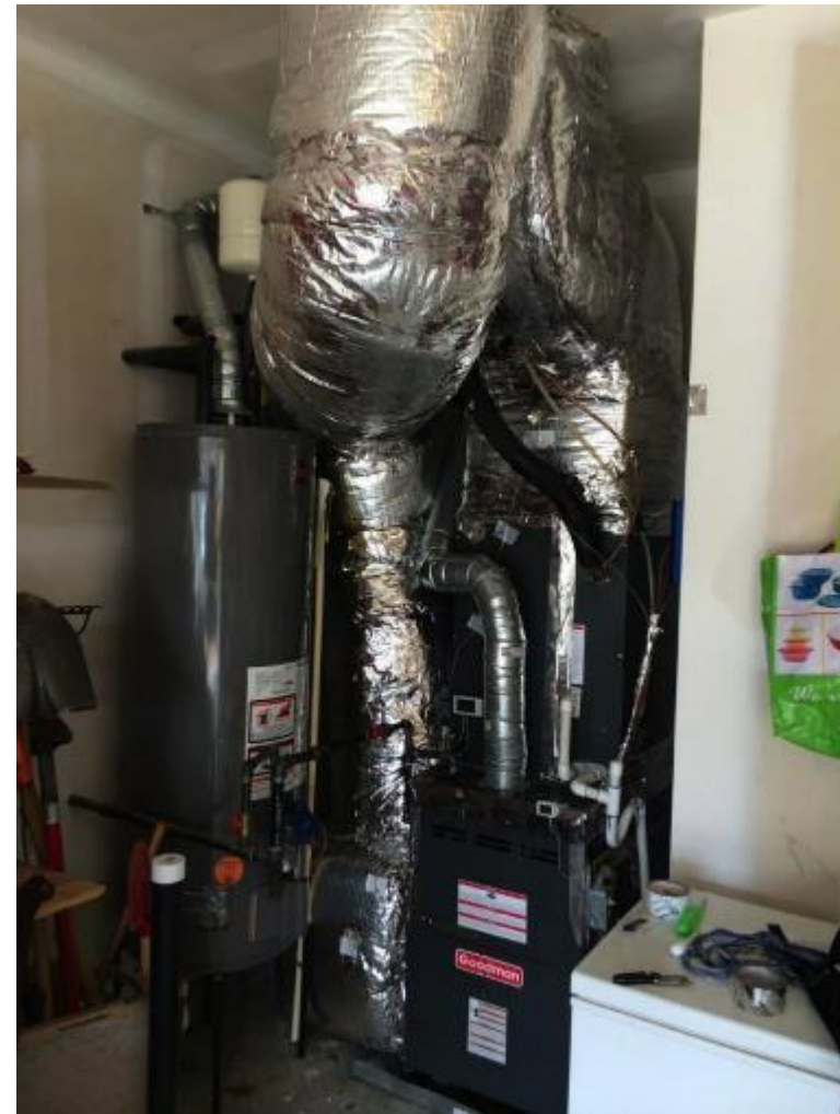
Picture Source: Construction Instruction
