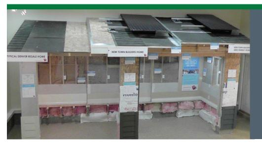
The building science center within the company's sales office compares New Town's advanced framing techniques, raised heel trusses, insulation, and air sealing with a typical Denver resale home. The buyer can actually see the difference between a high-performing zero-energy home and a typical existing home.
