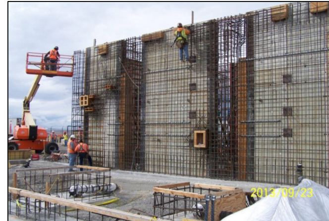
Construction of K-West Basin Annex for sludge retrieval project
