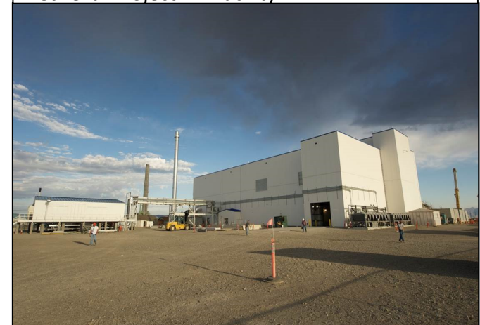
Integrated Waste Treatment Unit Facility
