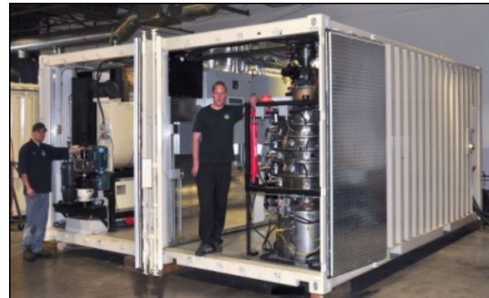
Community Power Corp: MEWEPS System
