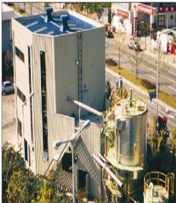
Two-phase thermophilic anaerobic digestion of MSW, Anyang City, S. Korea From CADDET Technical Brochure No. 66
