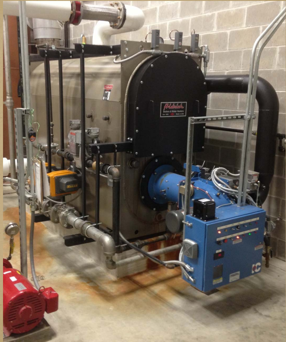
Dual Fuel Boiler
