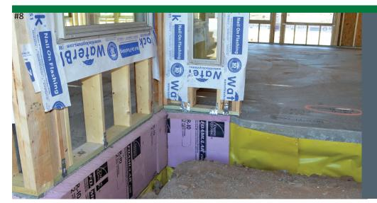
Two inches of rigid foam insulates the sides of the post-tensioned slab foundation. A 20-mil-thick plastic vapor barrier wraps the bottom and sides of the slab, preventing moisture from migrating from the ground into the concrete.
