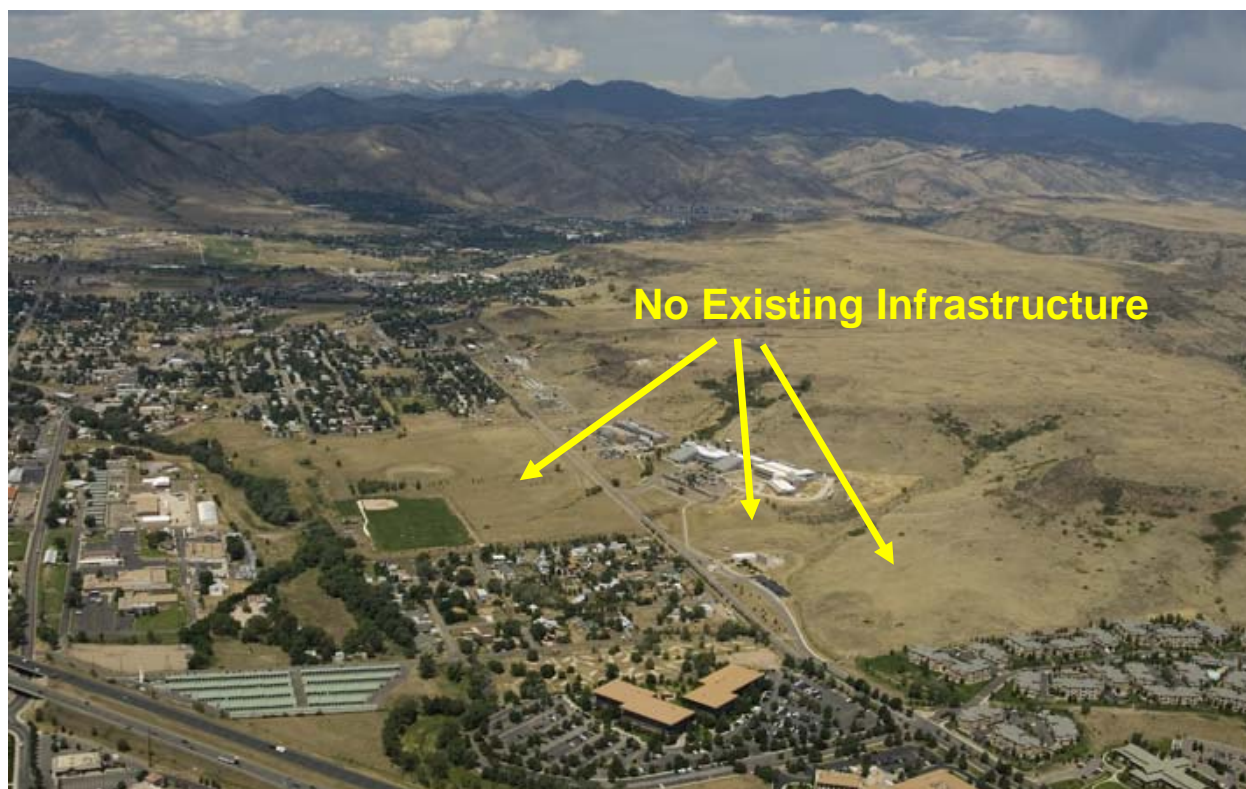
Figure 3.2.1. NREL's South Table Mountain campus buildout requires roads and utility
