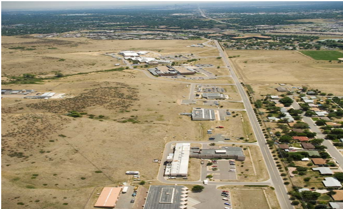
Figure F.5. South Table Mountain Site (looking from west)
