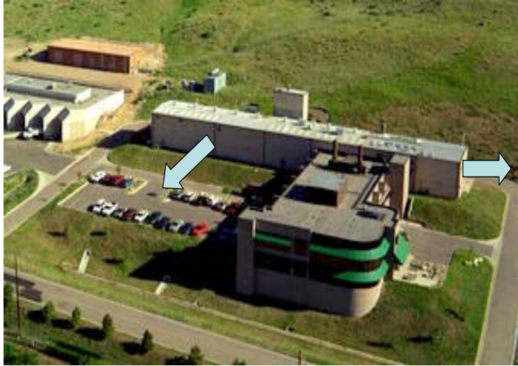
Figure 1.7.1 Integrated Biorefinery Research Facility Expansion. (Proposed expansion indicated by blue arrows).
