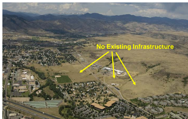
Figure 1.14.1 Major areas of NREL’s primary campus have no roads or utilities.
