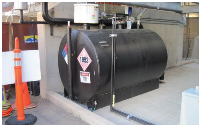
Diesel storage tank at the STM site. Photo by Larry Durbin, NREL 24478
