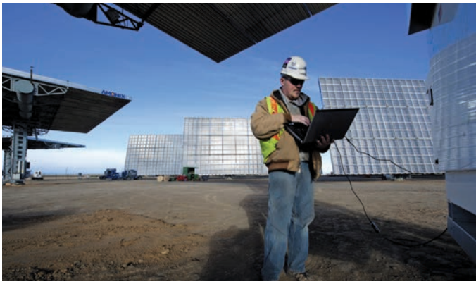
The SolarTAC test facility in Aurora, Colorado. Photo by Dennis Schroeder, NREL 19110
