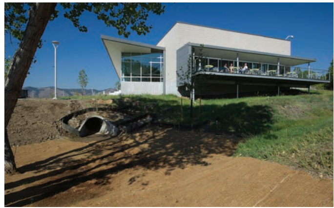
Stormwater erosion control matting at the cafeteria at the STM site. Photo by Dennis Schroeder, NREL 22488
