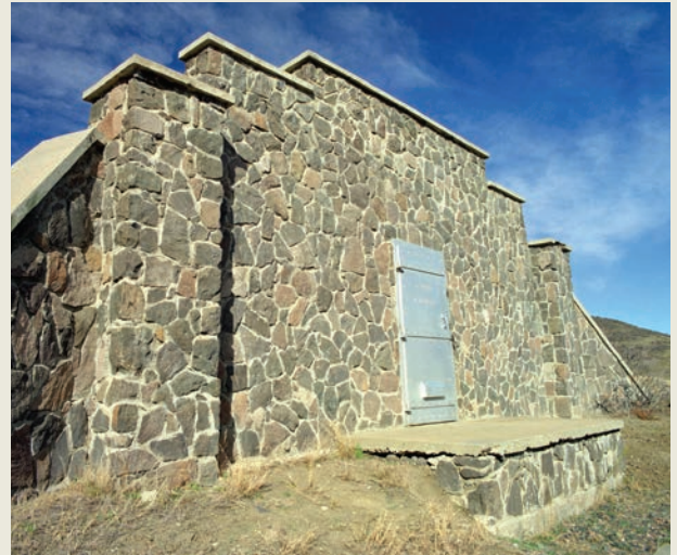
Ammo bunker constructed in 1940 at Camp George West. Photo by David Parsons, NREL 06928
