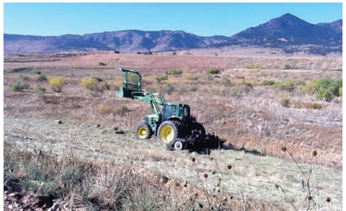
Reseeding and mulching following construction activity at NWTC. Photo by Genny Braus, NREL 24489
