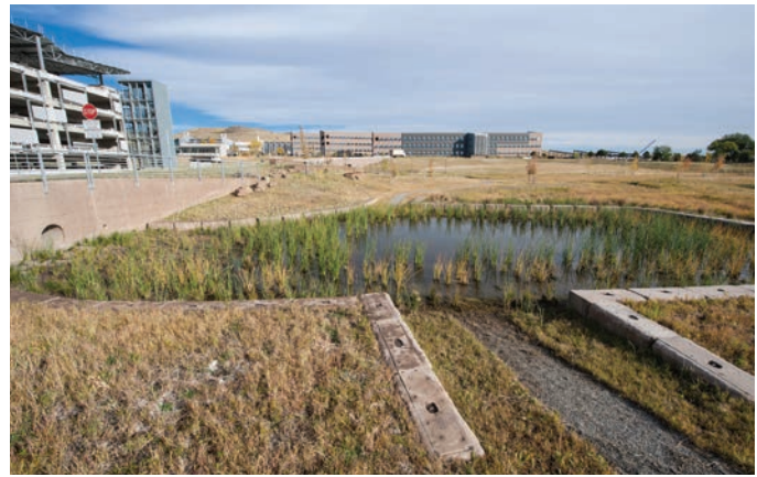
A new stormwater detention pond controls the flow of runoff from much of the STM site and serves as an important local habitat. Photo by Dennis Schroeder, NREL 23195
