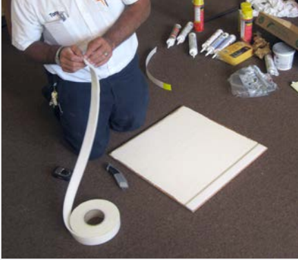
Gaskets and insulation were added to attic hatches.
