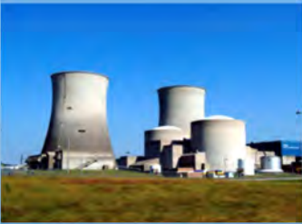
Watts Bar Nuclear Plant
