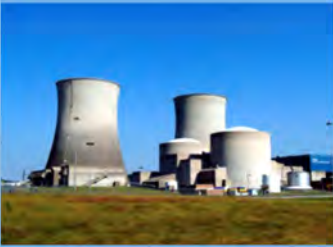
Watts Bar Nuclear Plant
