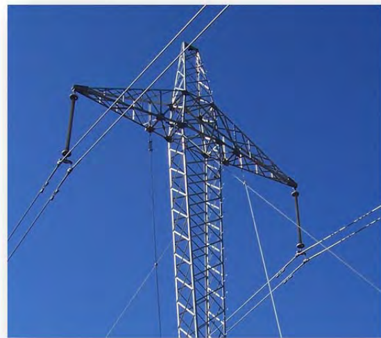
Figure 2.1-7: Glass Insulators on Dead-end and Rigid Insulators on Guyed Tower
