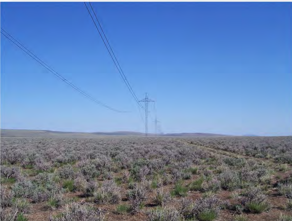
Figure 3.9-3: Shrubland near Tower 207/5
