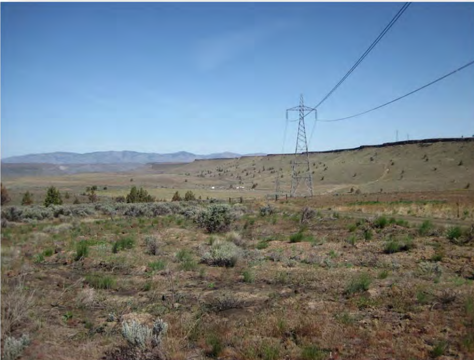
Figure 3.9-2: Transmission Line Crossing of US 97 at Tower 61/1
