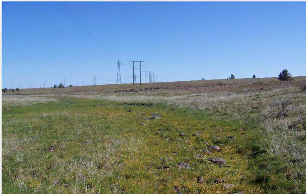
Figure 2.1-3: Existing PDCI Line North of US 97-US 197 Intersection (looking north from Tower 48/1, Big Eddy-Redmond No 1 is on the right)
