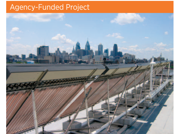
Agency-Funded Project Social Security Administration, high-temperature hot water project, Philadelphia, Pennsylvania, 54-m 2 solar thermal system
