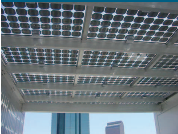
Alfred A. Arraj U.S. Courthouse; Denver Federal Courthouse; PV system supplied by Atlantis Energy Systems PV shade structure on the top floor is cantilevered over facade; first federal courthouse to get PV glazing. (Credit: Atlantis Energy Systems, Inc., PIX 13999)
