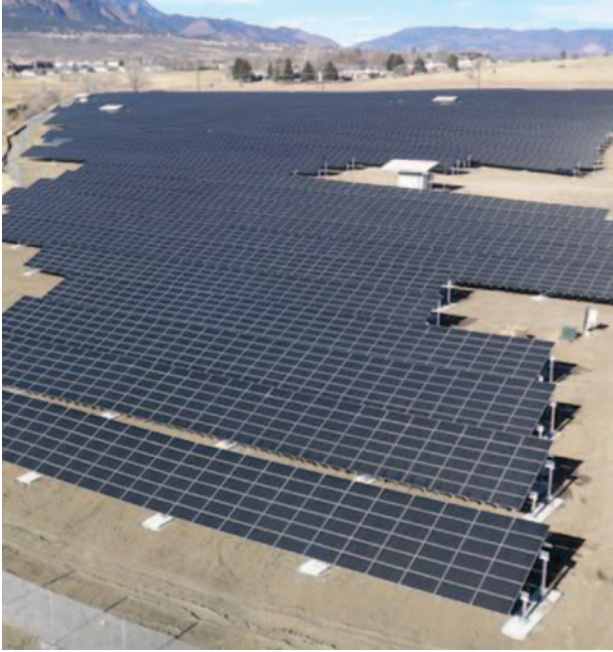
Fort Carson PV Project, Colorado Springs, Colorado, 2-MW PV (Credit: U.S. Army Fort Carson. PIX 17394.)
