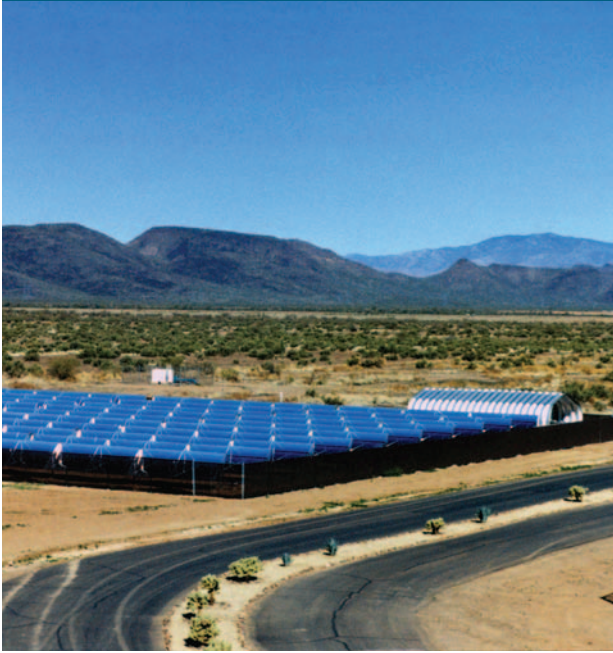
Phoenix Federal Correctional Institution, Phoenix, Arizona, parabolic trough solar water-heating system. (Credit: Ed Hancock, Mountain Energy Partnership. PIX 09048.)
