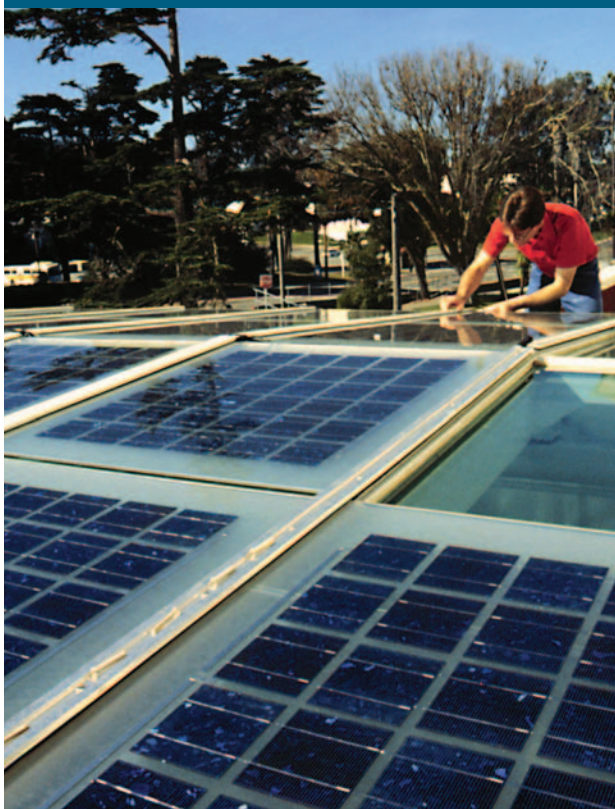
Installation of skylight glass laminated with PV cells at the Thoreau Center for Sustainable Development, Presidio National Park, San Francisco, California.. (Credit: Lawrence Berkeley Lab, PIX 01056)
