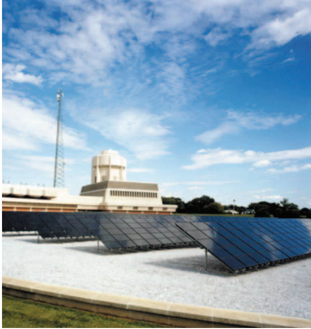
Suitland Federal Center PV system, Maryland. (Credit: Bob Madani for DOE/FEMP. PIX 10726.)
