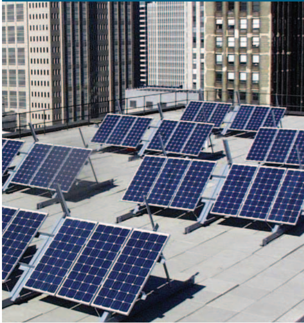
General Services Administration, Ralph H. Metcalfe Federal Building PV arrays, Chicago, Illinois. (Credit: Patrick Engineering. PIX 09514)
