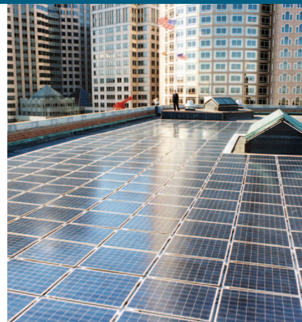
United States Coast Guard – The Williams Building in downtown Boston, Massachusetts, now has a 28 kW AC PV system integrated into the roof consisting of 372 panels. (Credit: SunPower, PIX 08466)
