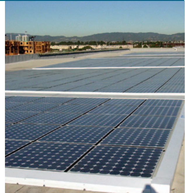
PV solar array installed at Marina Del Rey USPS Postal Station in Los Angeles, California. (Credit: George Marsh, PIX 11015)
