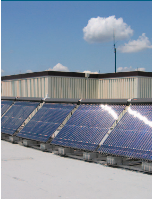
Social Security Administration, high-temperature hot water project, Philadelphia, Pennsylvania, 54-m 2 solar thermal system (Credit: Ed Hancock, Mountain Energy Partnership)
