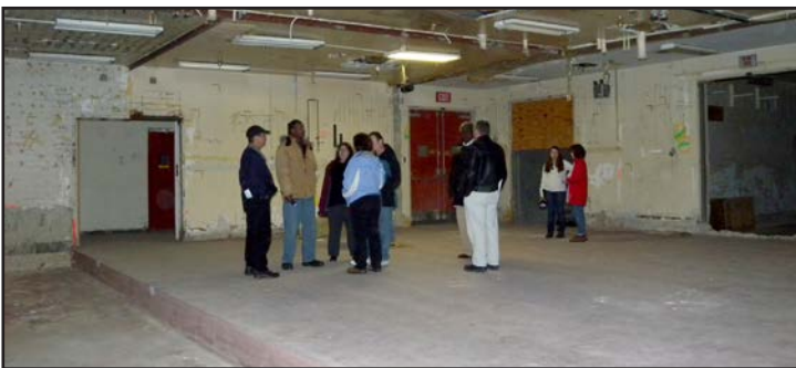
The annual institutional controls assessment at the Mound site includes interviews with property owners; reviews of local, county, and state records; and a physical walkdown of the site and buildings.
