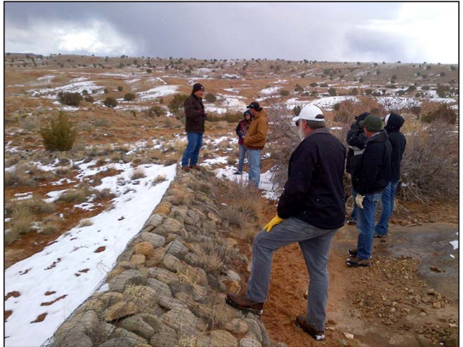
Gilbert Dayzie, Navajo Nation AML civil engineer, describes the flow-through design of rock-lined diversion berms to LM representatives.
