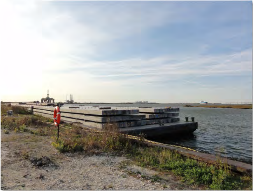
Piles Arriving by Barge (10-Dec-2012)
