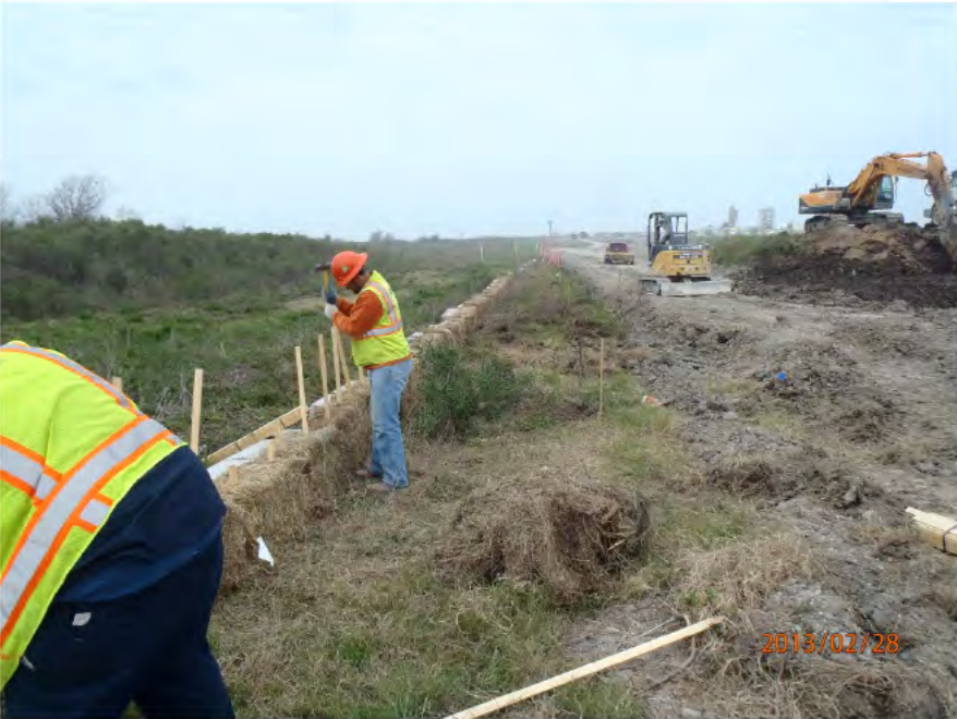
Reinforced hay bales installed along Heavy Haul Road (28-Feb-2013)
