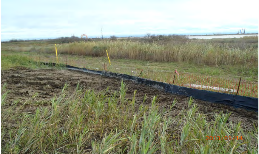
Silt fence installation between the Ro-Ro and the pipeline bridges (14-Jan-2013)
