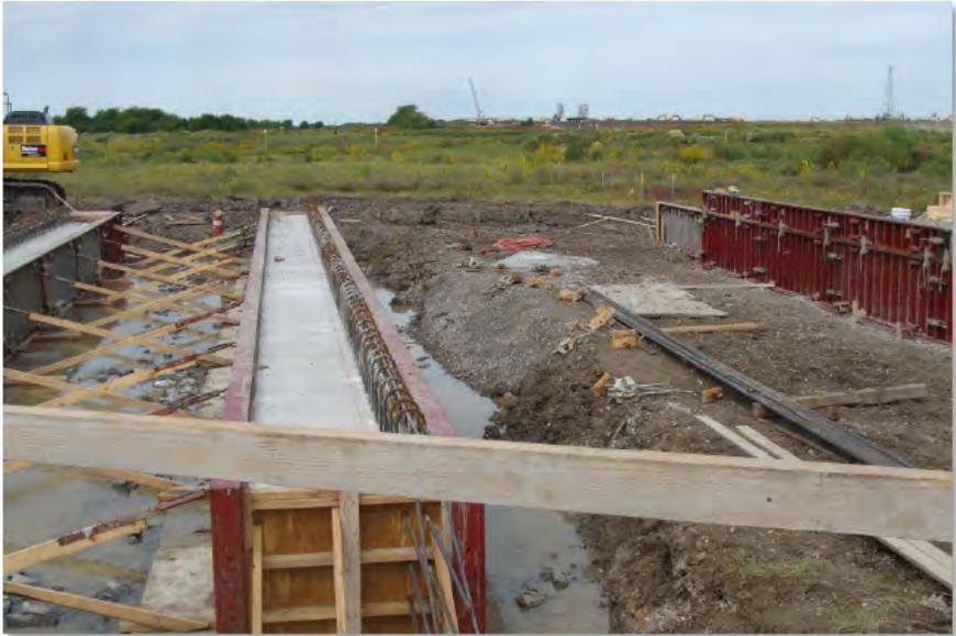
Heavy Haul Road Pipeline Bridge Crossing (18-Oct-2012)
