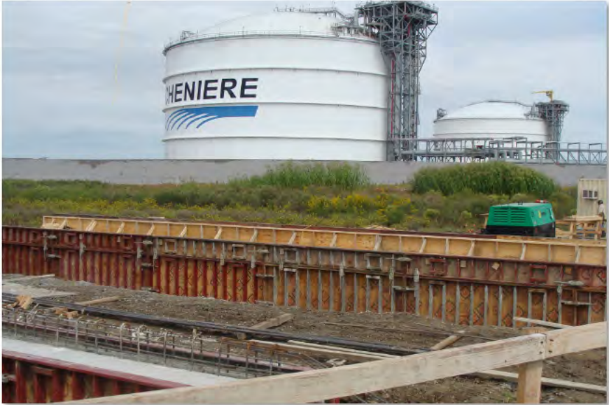
Heavy Haul Road Pipeline Bridge Crossing (18-Oct-2012)
