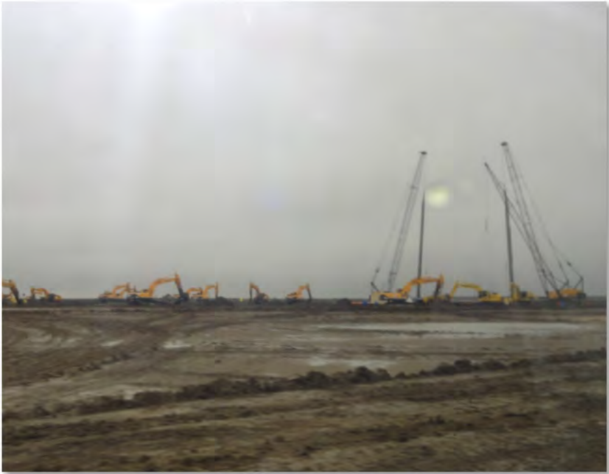
Train 1 / Train 2 Mixing (27-Nov-2012)
