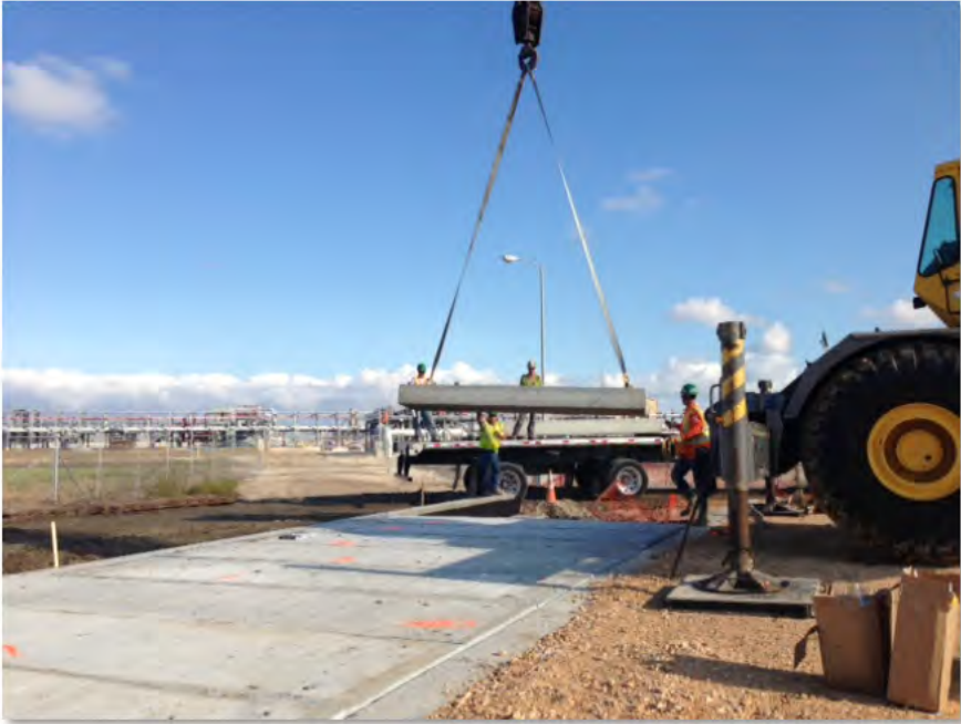
Pipeline Crossing Bridge Panel Installation (05-Dec-2012)
