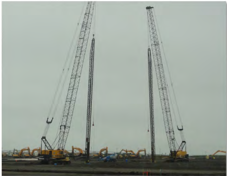
Train 2 Soil Mixing (27-Nov-2012)
