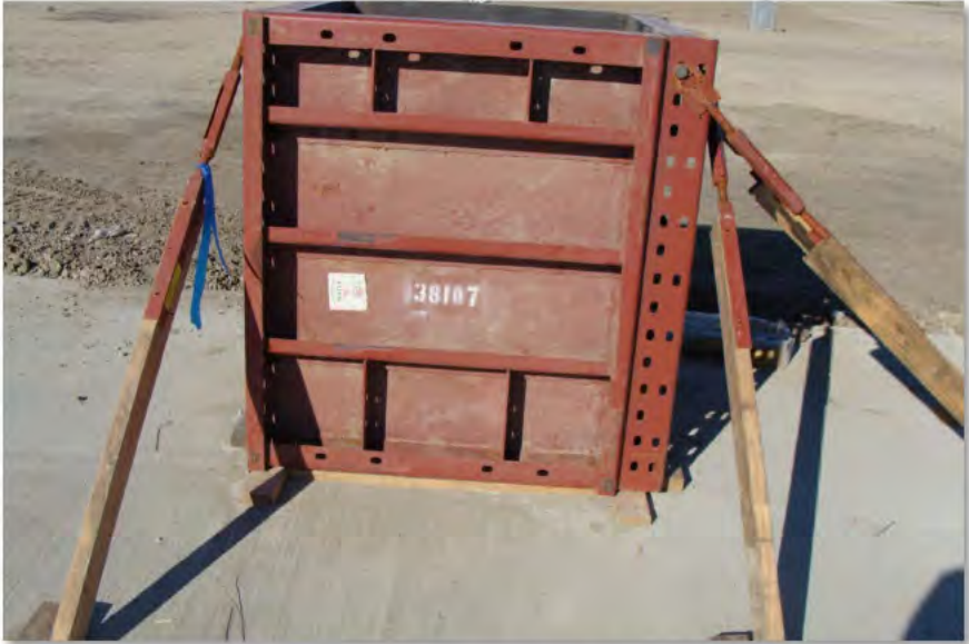
Pedestal Formwork (14-Feb-2013)
