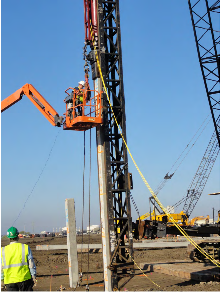
Pile Drive Analyzer (28-Nov-2012)
