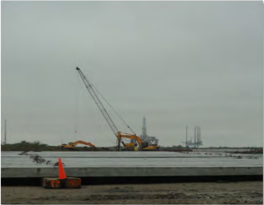
Pile Laydown near the Construction Dock (27-Nov-2012)
