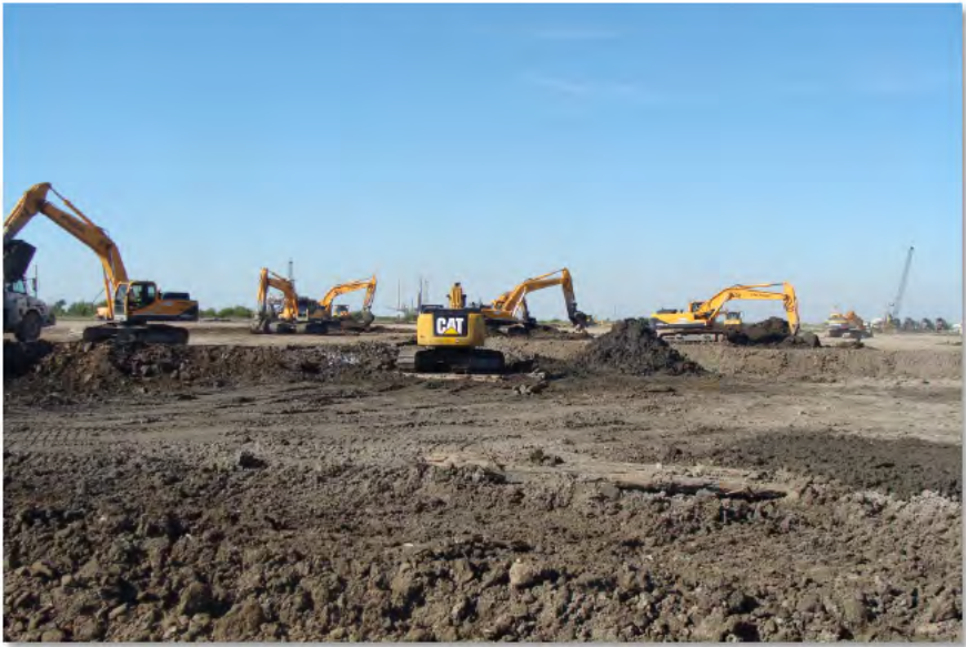
Recon Excavators Improving Soil (30-Oct-2012)
