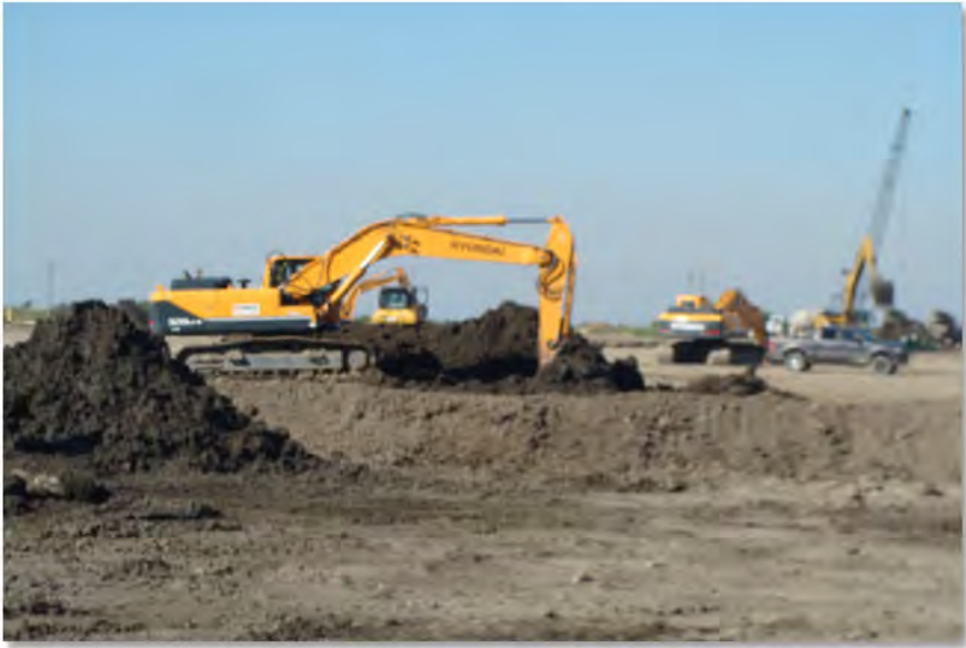
Recon Excavators Improving Soil (30-Oct-2012)
