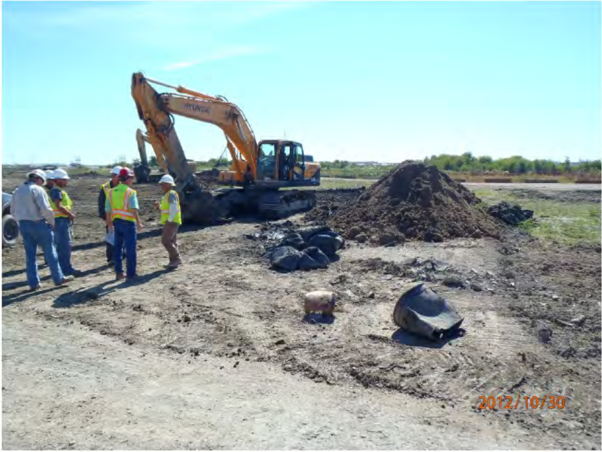
Waste drums uncovered during soil prep (30-Oct-2012)
