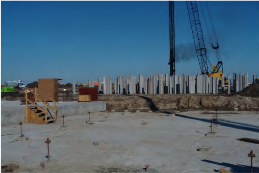
Pile Tension Connectors 131N (14-Feb-2013)
