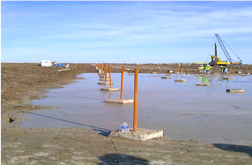
Pile Tension Connectors in Area 131N (14-Jan-2013)
