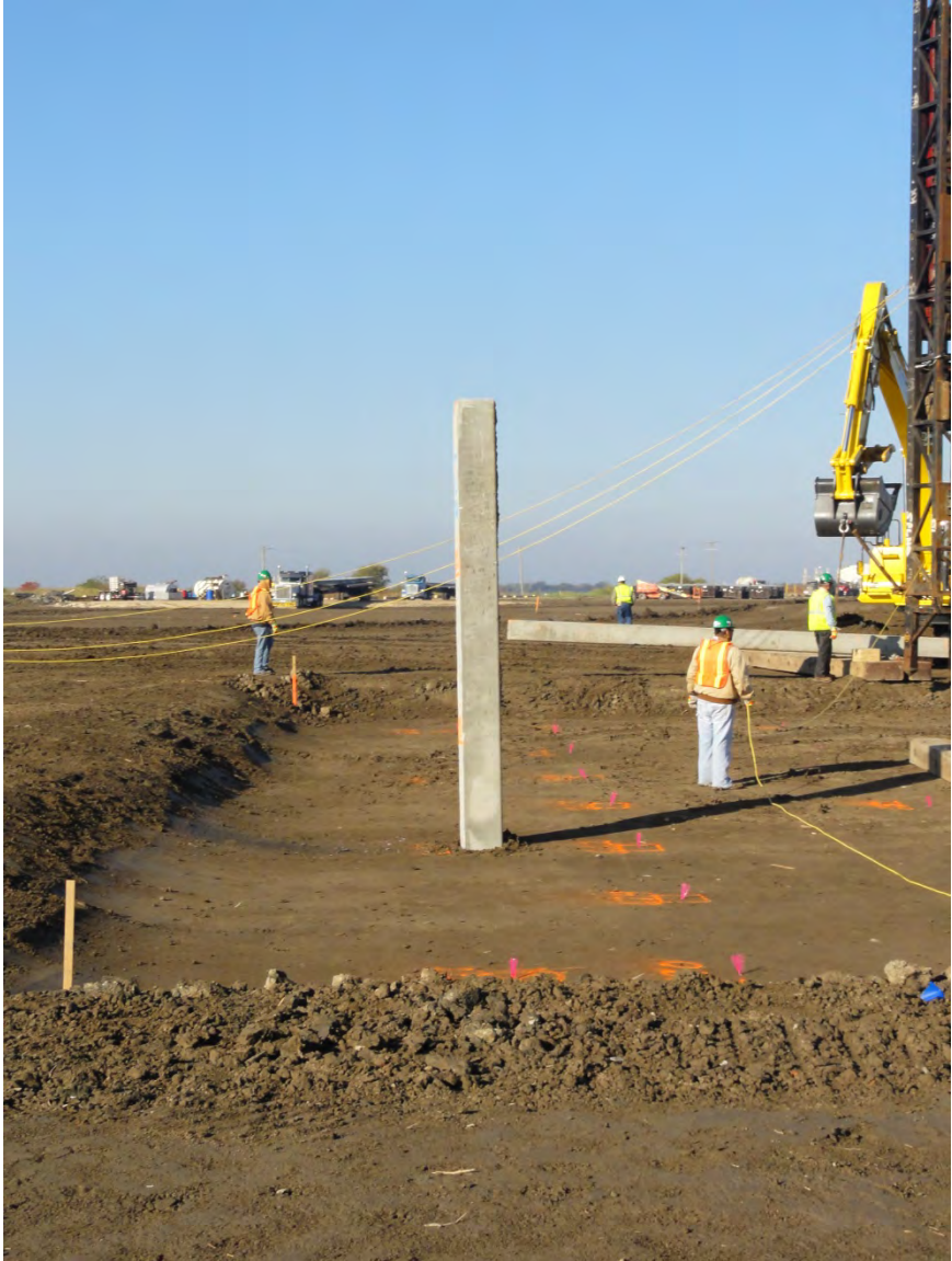
First Pile (28-Nov-2012)
