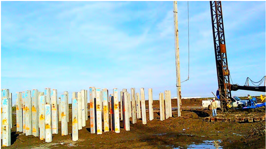
Pile Driving, Area 131N (14-Jan-2013)
