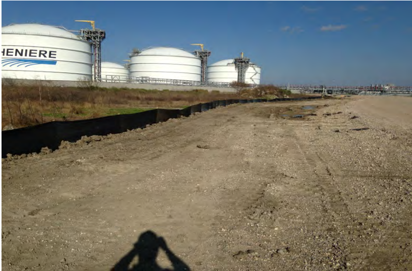
Installation of silt fence near the low pressure vent stack (14-Jan-2013)
