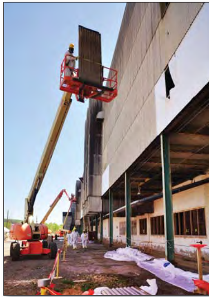
Workers remove panels from the K-31 Building in preparation for demolition.
