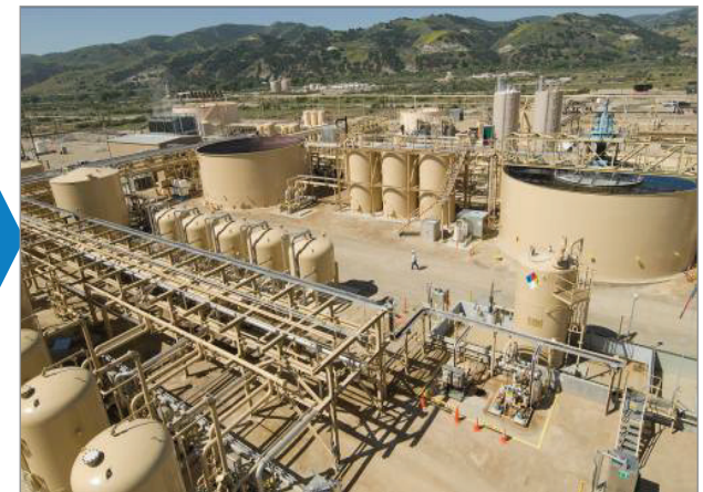
Veolia produced water treatment plant
