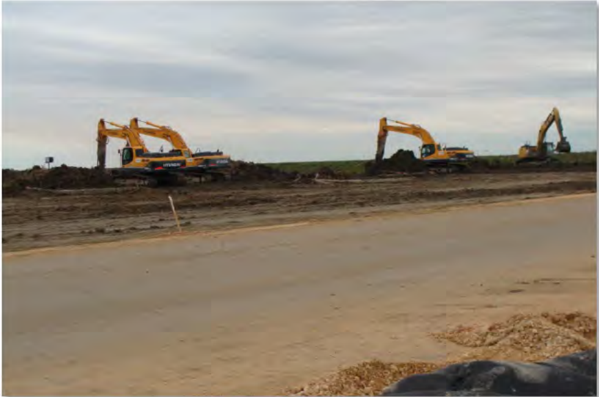
Road Work and Soil Mixing, Recon (14-Feb-2013)
