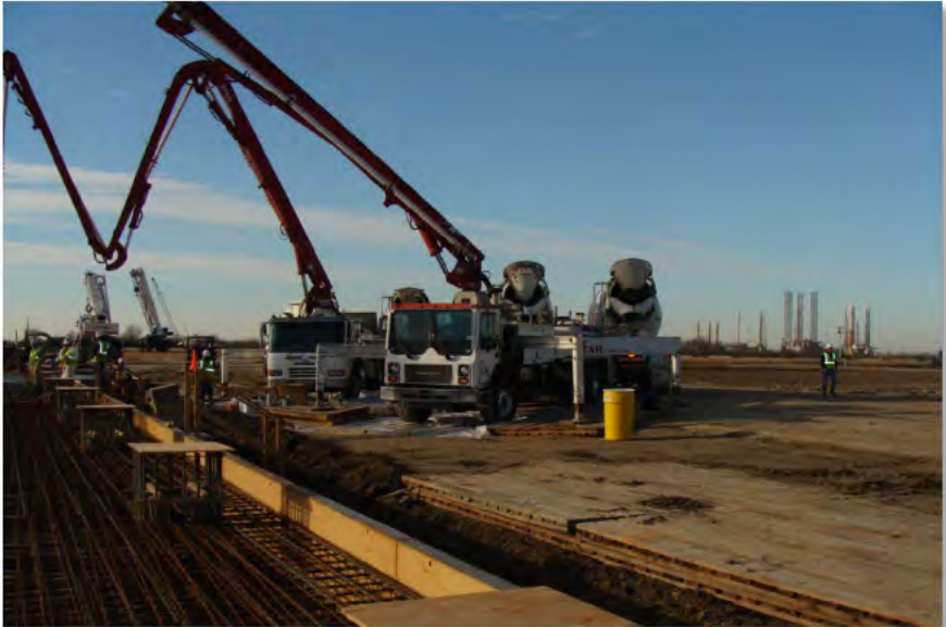
Concrete Pump Trucks (14-Feb-2013)
