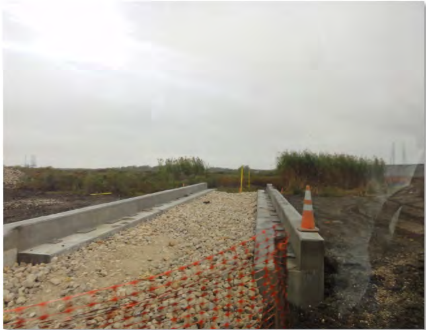
Pipe Bridge ready for Top Panels (27-Nov-2012)
