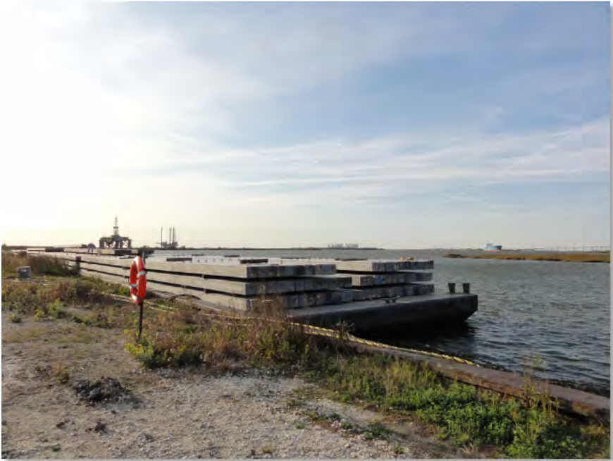
Piles Arriving by Barge (10-Dec-2012)
