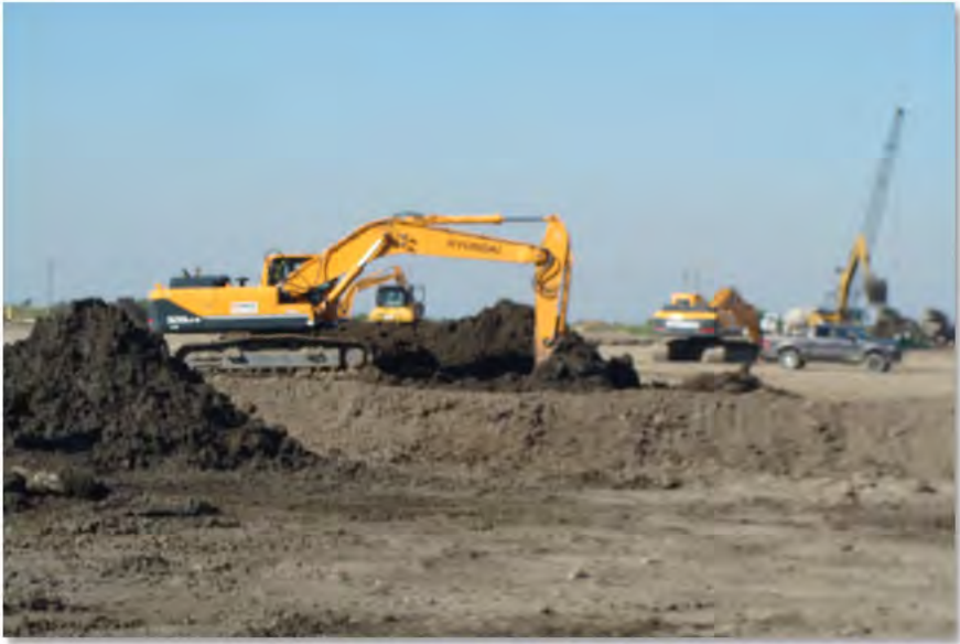
Recon Excavators Improving Soil (30-Oct-2012)
