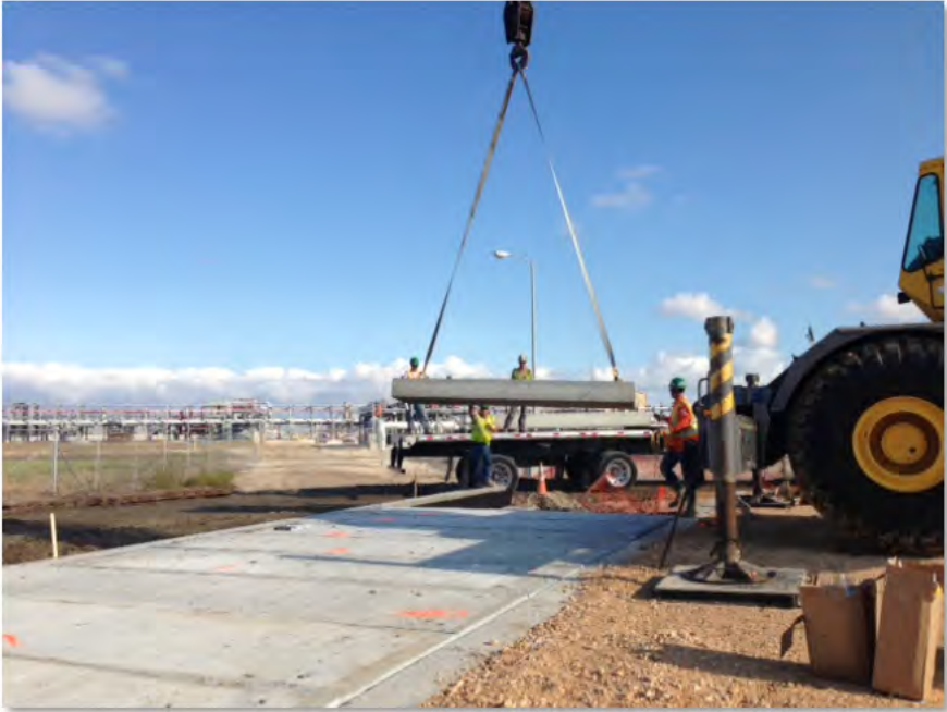
Pipeline Crossing Bridge Panel Installation (05-Dec-2012)
