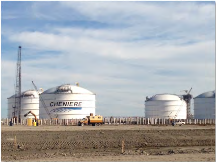
Piling Progress in Area N (21-Dec-2012)
