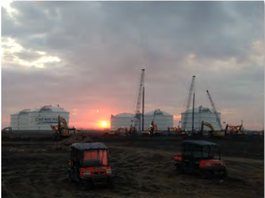
Piling Progress in Area N (21-Dec-2012)
