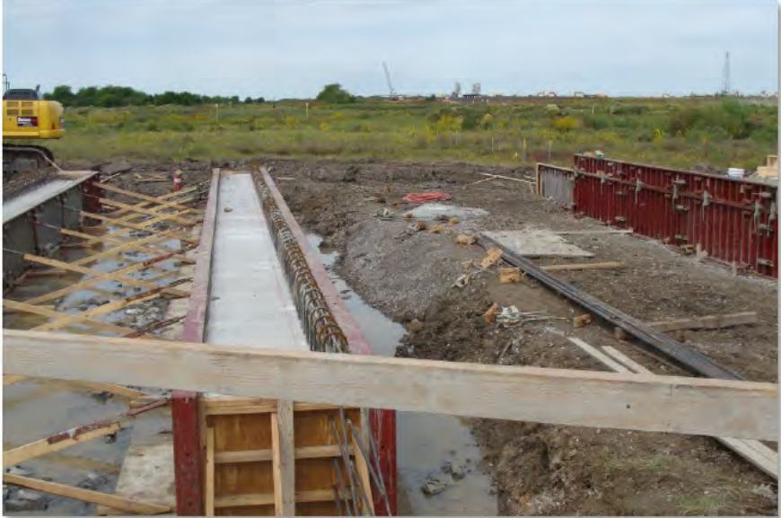
Heavy Haul Road Pipeline Bridge Crossing (18-Oct-2012)
