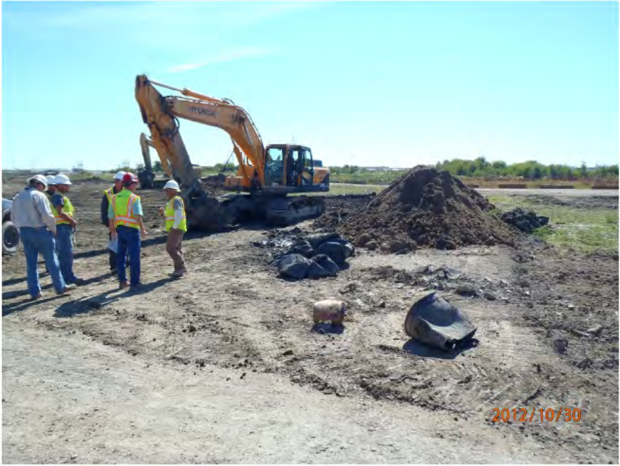
Waste drums uncovered during soil prep (30-Oct-2012)
