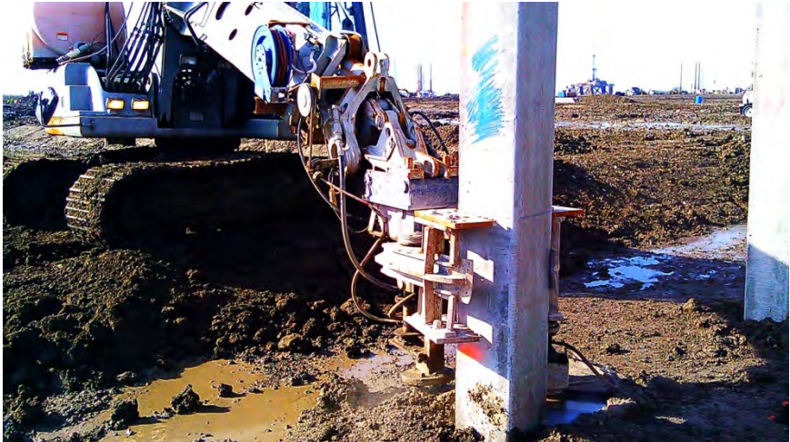
Pile Cutting in Area 131N (14-Jan-2013)
