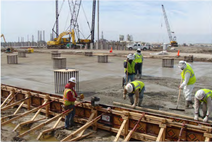
Finishing the Pour, 131N (14-Feb-2013)
