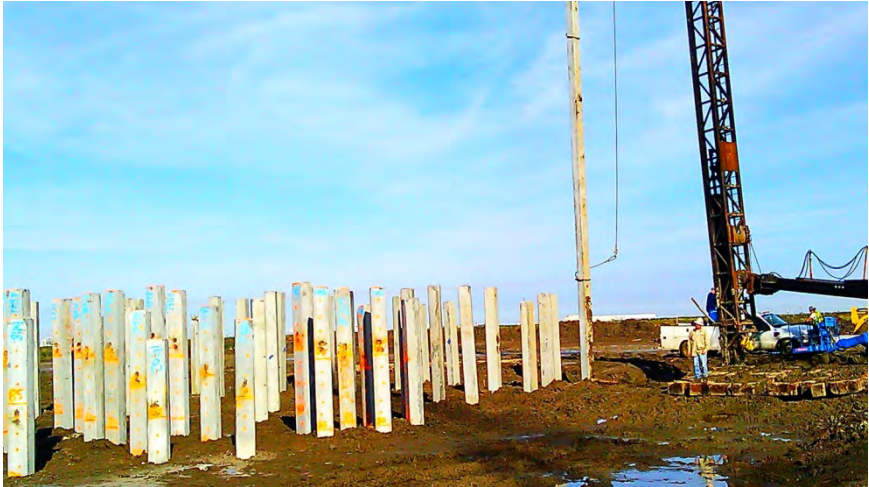
Pile Driving, Area 131N (14-Jan-2013)
