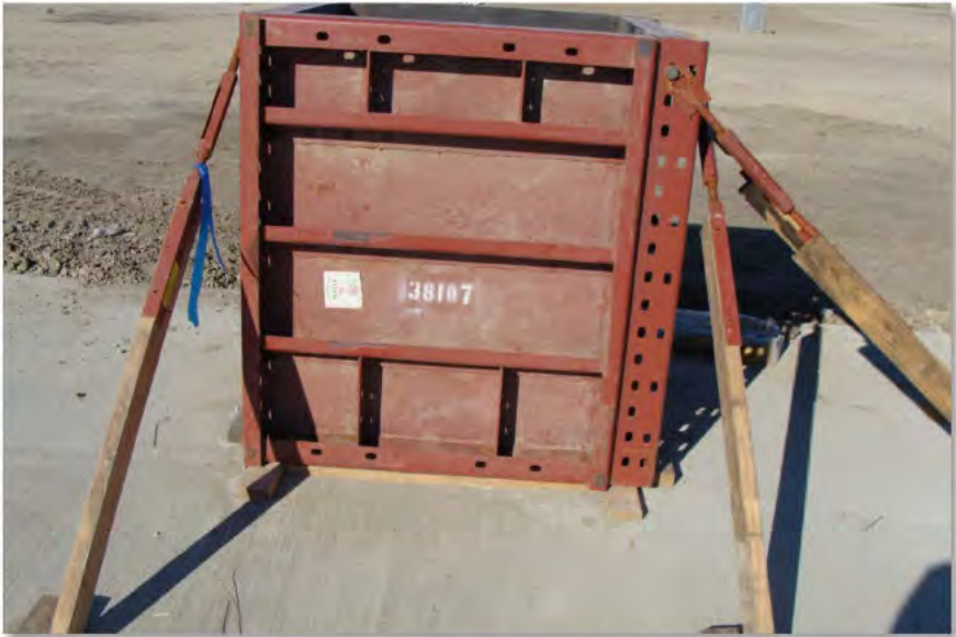
Pedestal Formwork (14-Feb-2013)
