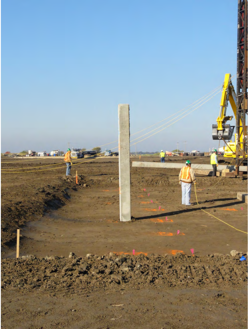
First Pile (28-Nov-2012)
