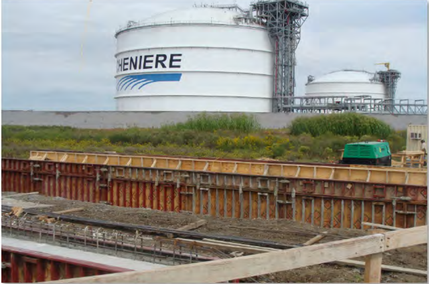
Heavy Haul Road Pipeline Bridge Crossing (18-Oct-2012)
