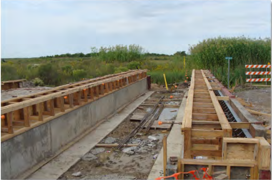
Heavy Haul Road Pipeline Bridge Crossing (18-Oct-2012)
