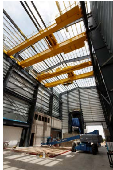
5 MW Building Construction
