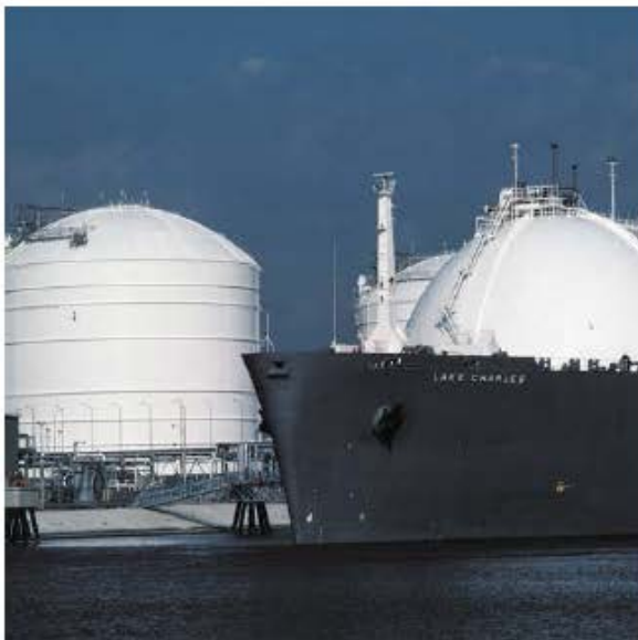
The liquefied natural gas storage tanks at the existing Lake Charles LNG facility.
