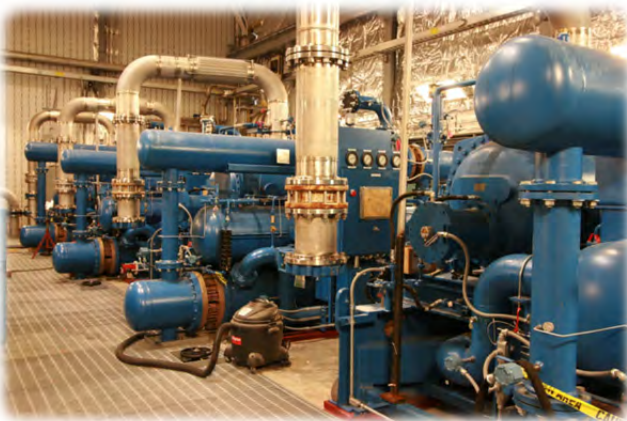
Figure 3-10 Cryogenic Plant Compressor Room
