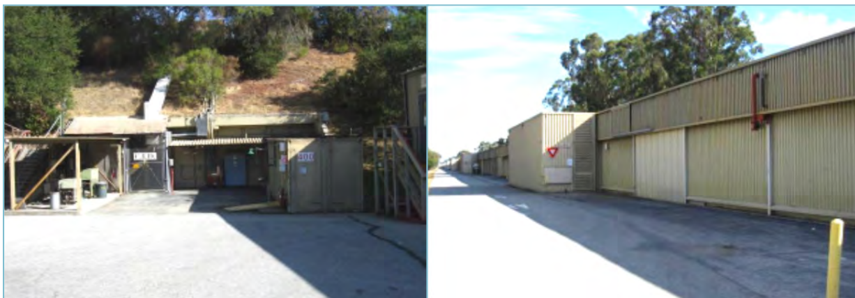
Figure 3-3 Existing Structures in the Project Area (Building 001-Accelerator Housing [entrance shown at left] and Building 002: Klystron Gallery [right])
