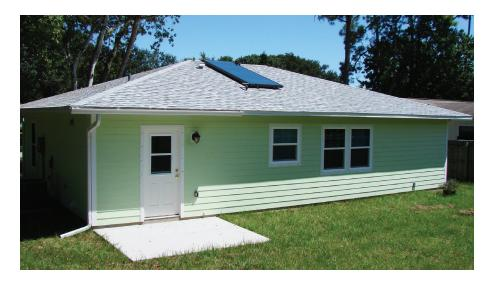
Solar thermal panels, mounted on the south-facing rear roof, provide plenty of hot water at a cost of only \$121 a year to run, compared to \$282 a year for a conventional 80-gallon, 89%-efficient water heater.
