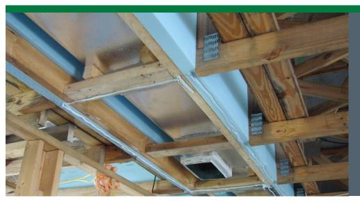
After the rigid foam sides were installed, the rectangular fiberboard duct was lifted into place and supported with 2x4 blocking. Most of the duct registers came directly off the main trunk and boots were installed before raising the duct. The rigid foam chase was further covered with R-11 of unfaced batt for a total chase insulation value of R-31. After the ceiling drywall was installed, R-38 of blown cellulose was blown onto the attic floor around the chase.
