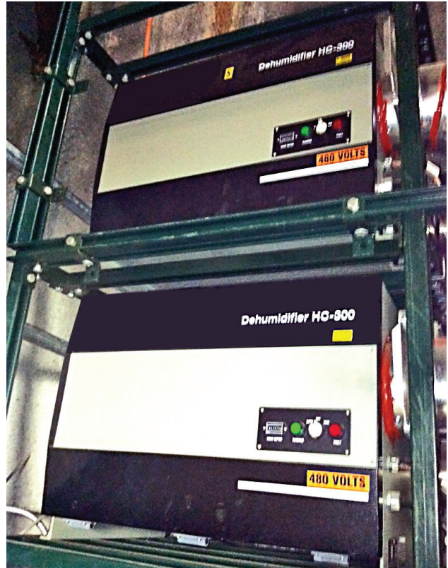
Exhibit 4-8: NuMI Dehumidification Units
