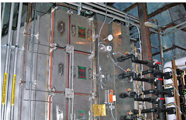
Exhibit 4-10: NuMI Target Hall Ventilation Bank
