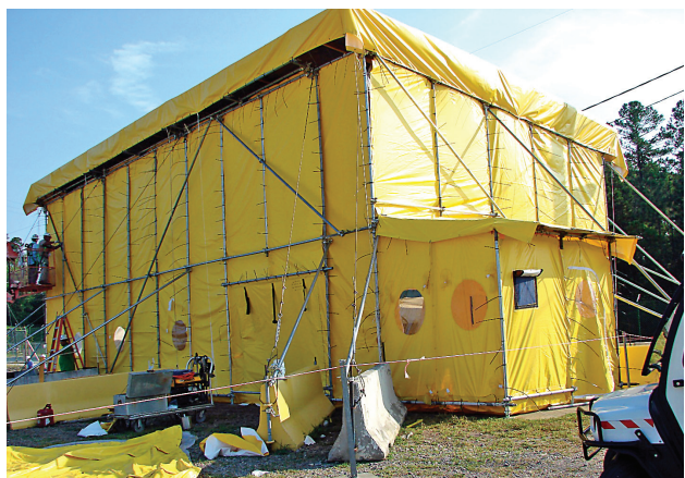
Exhibit 4-15: Containment Hut with HVAC System
