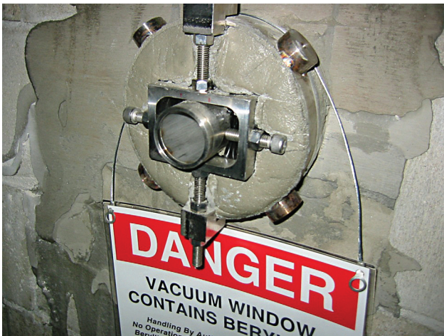
Exhibit 4-9: NuMI Beryllium Window Vacuum Pipe Removal
