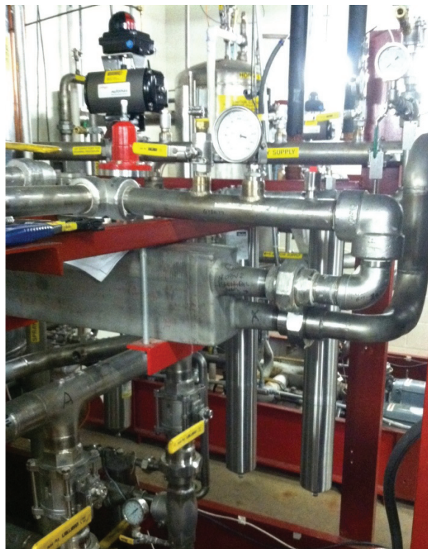
Exhibit 4-6: NuMI Radioactive Water Piping
