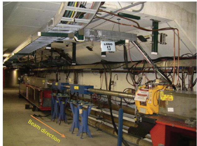
Exhibit 4-5: Booster Notching Absorber
