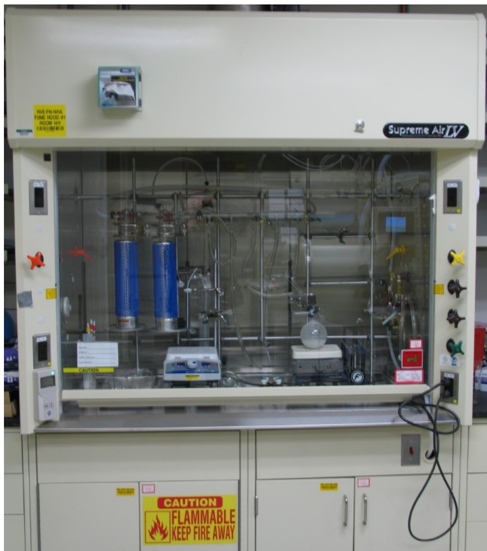
Low Flow Type Chemical Fume Hood with VAV
