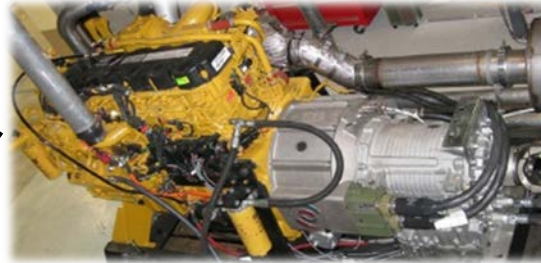
Engine w/ Generator
