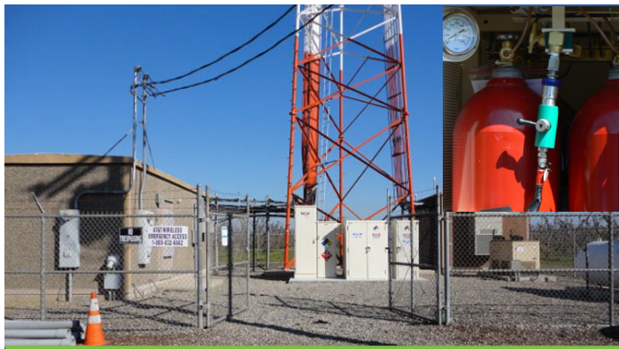
Refueling hydrogen tanks for backup power (top right); AT&T cellular tower site with fuel cells for backup power. ReliOn, Inc.
