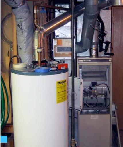
For existing systems in the basement of a single-family home, space heat was provided by a forced-air natural gas furnace with an AFUE rating of 78%. Water heating was provided by a natural draft natural gas water heater with an EF rating of 59%.
