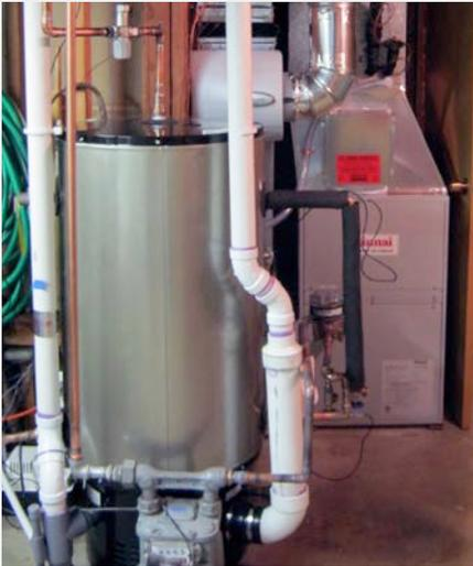
This photo shows a combi system replacement using a condensing storage water heater and a hydronic air handler. At this home, this system saved more than 20% on space and water heating natural gas usage.
