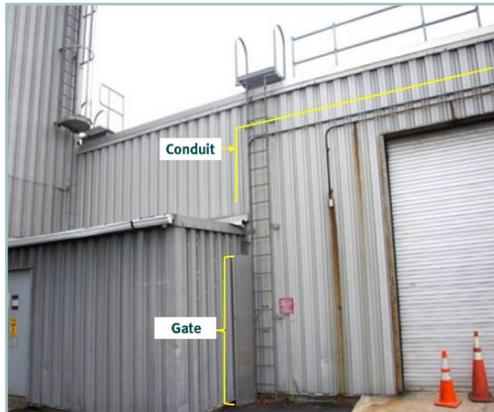
**Figure 2-1. Current location of the fixed ladder showing gate and conduit**
