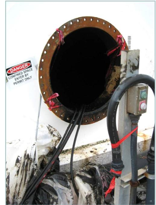
**Figure 2-3. Tank opening for workers' ingress/egress (posted as Confined Space)**
