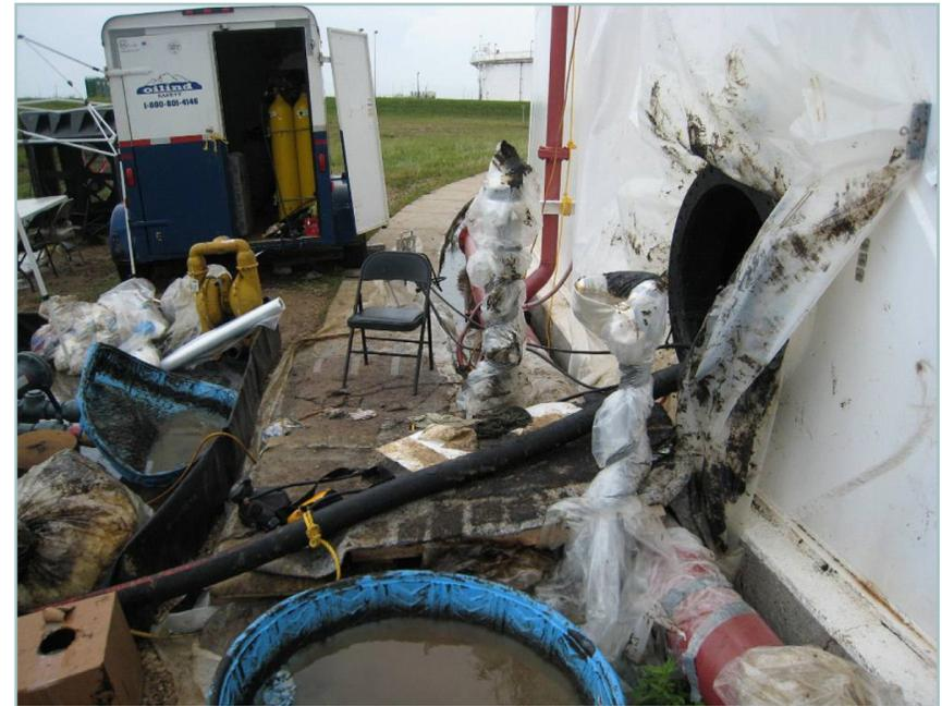
**Figure 2-4. Tank opening used by the subcontractor to feed air hoses to workers inside tank**
