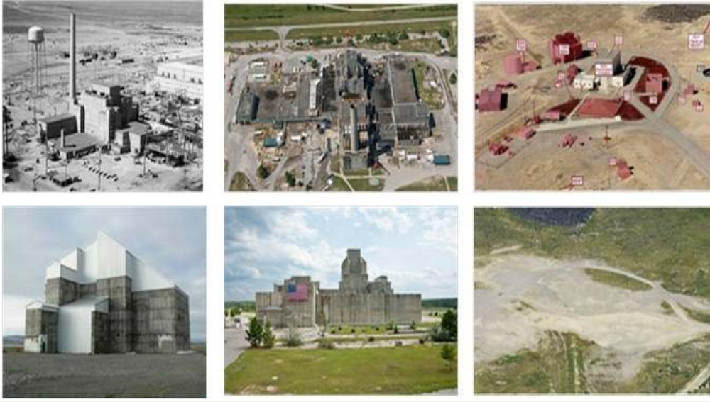
Three different D&D end states for reactors: (From left to right) interim stabilization at Hanford, in-situ decommissioning at SRS, and complete reactor removal at Idaho
