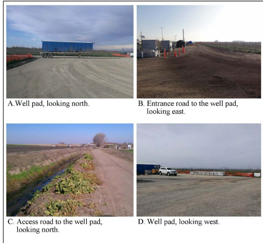
Figure 2-4. Views of and around the site.
