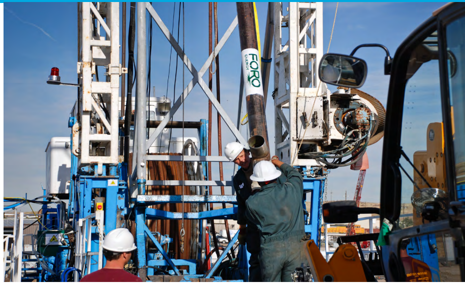
Foro Energy, Inc. partners with the United States Department of Energy (DOE) to commercialize high power lasers for the oil, natural gas, geothermal, and mining industries. Photo courtesy of Foro Energy
