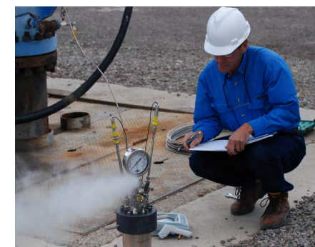
Flow test at the Faulkner plant in Nevada (top left); water vapor; DOE field testing.
