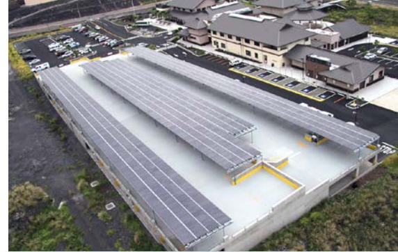
Hawai'i's government is embracing renewable energy technologies and leading by example, as shown in this photo of the West Hawai'i Civic Center (background), with its 250-kW solar PV array (foreground). Photo from Drew Bradley, REC Solar
