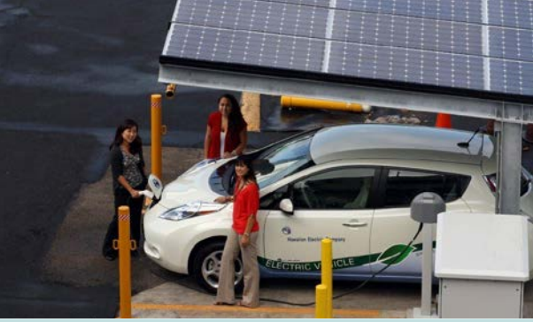
From sun to run: PV solar panels power an EV at a HECO carport charging station. Photo from HECO
