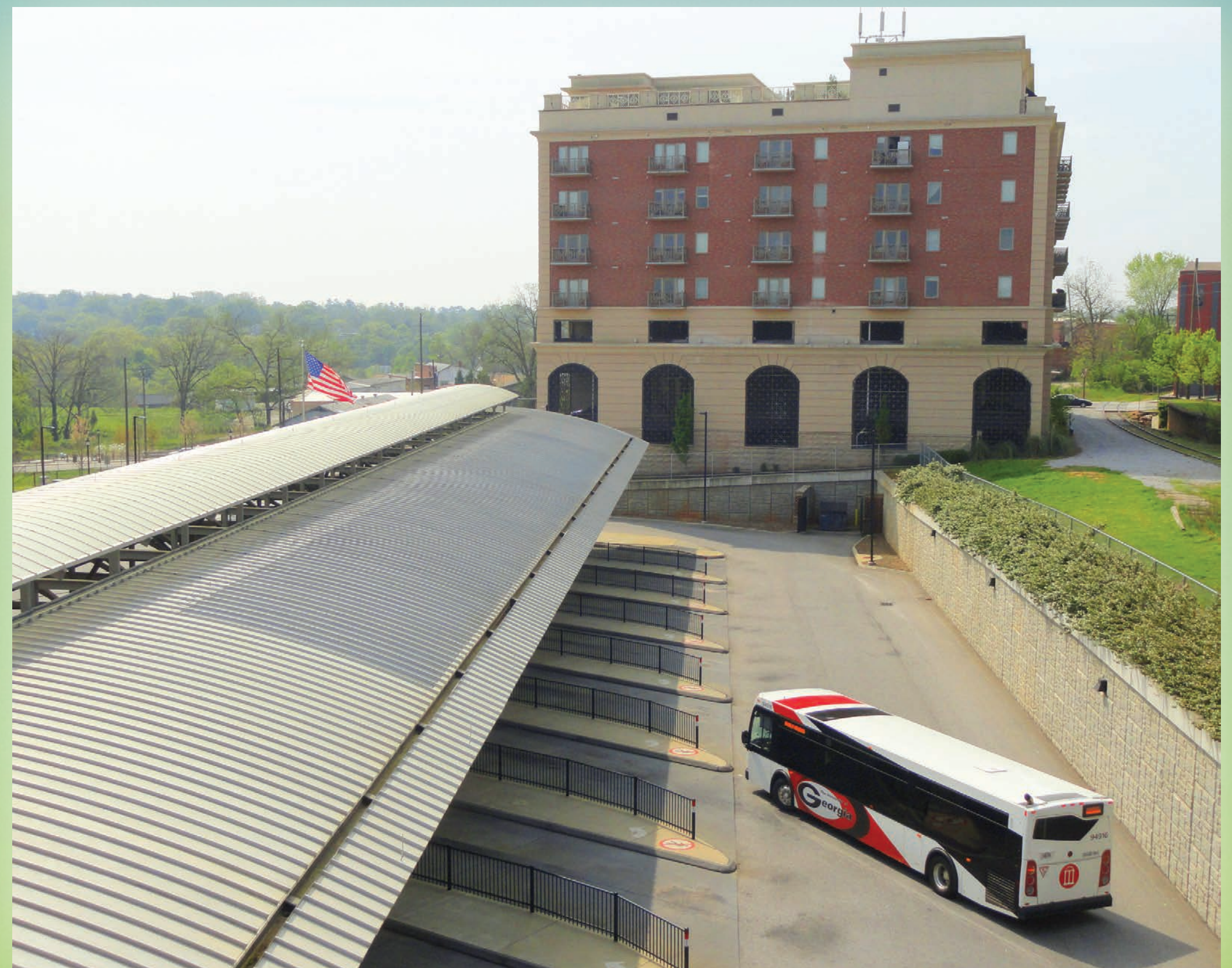
ENERGY EFFICIENCY: "Roof-Mounted Photovoltaic System" by Gary Hartman
