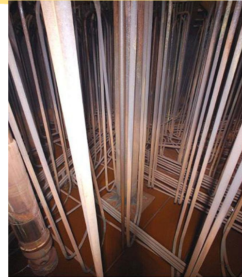
Savannah River Tank 5 Heel Removal (Tank Interior)
