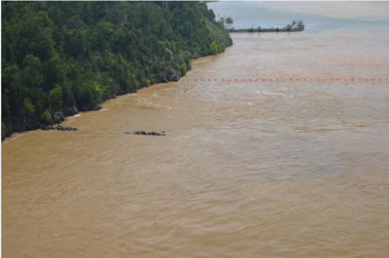
View looking downstream at diversion structure from top of spillway after gate test 3.
