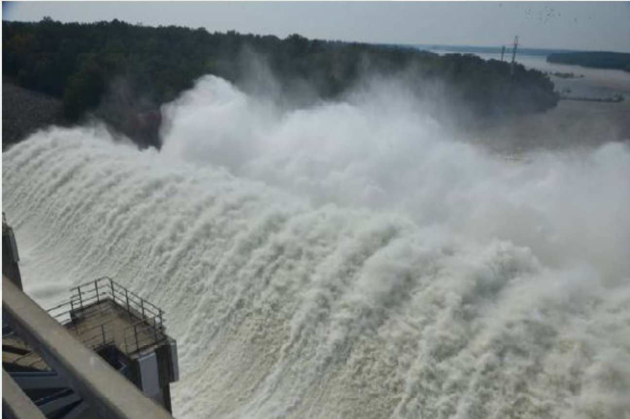
View looking downstream from top of spillway at gate 4 during second portion of gate test 2. Gates 1-3 opened 9 steps (7ft), gates 4-10 opened 5 steps (3.7ft).
