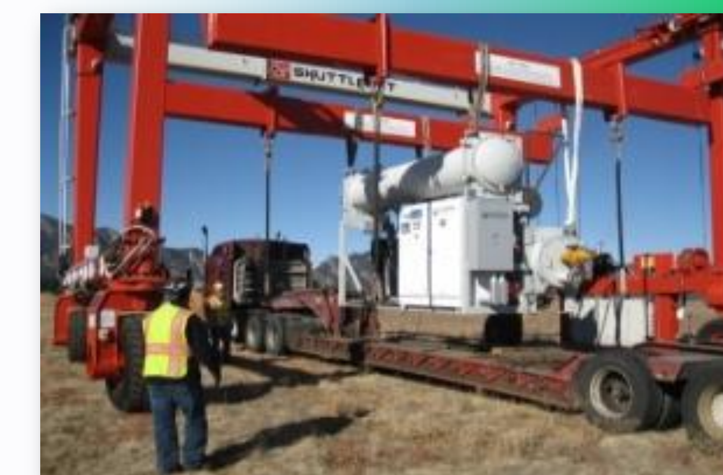
The Rocky Mountain Oilfield Testing Center (RMOTC) Relocation Project is designed to reduce the risks associated with co-production by operating binary units in commercial oil and/or gas fields. Technical site data will be collected to significantly reduce cost and performance uncertainties and lower the barrier for market uptake.
