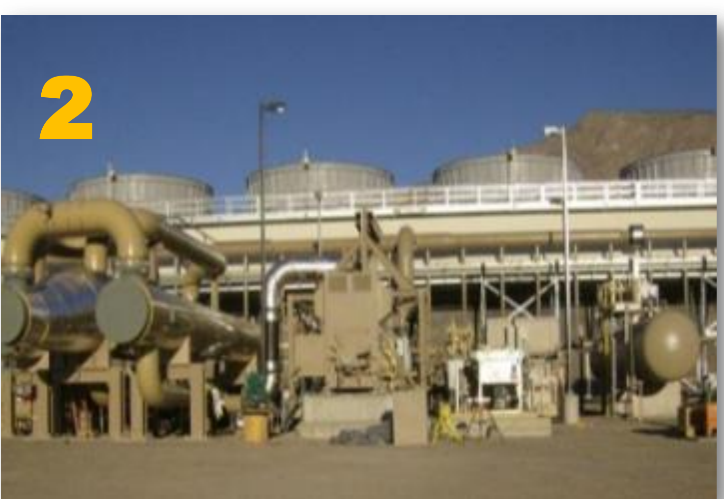
Terra-Gen at Dixie Valley is demonstrating the technical and economic feasibility of nonconventional geothermal resources (223°F), employing the first commercial use of a supercritical cycle at a geothermal power plant inlet temperature of less than 300°F. Since September 2012, the plant has been online and producing 6 MW.
