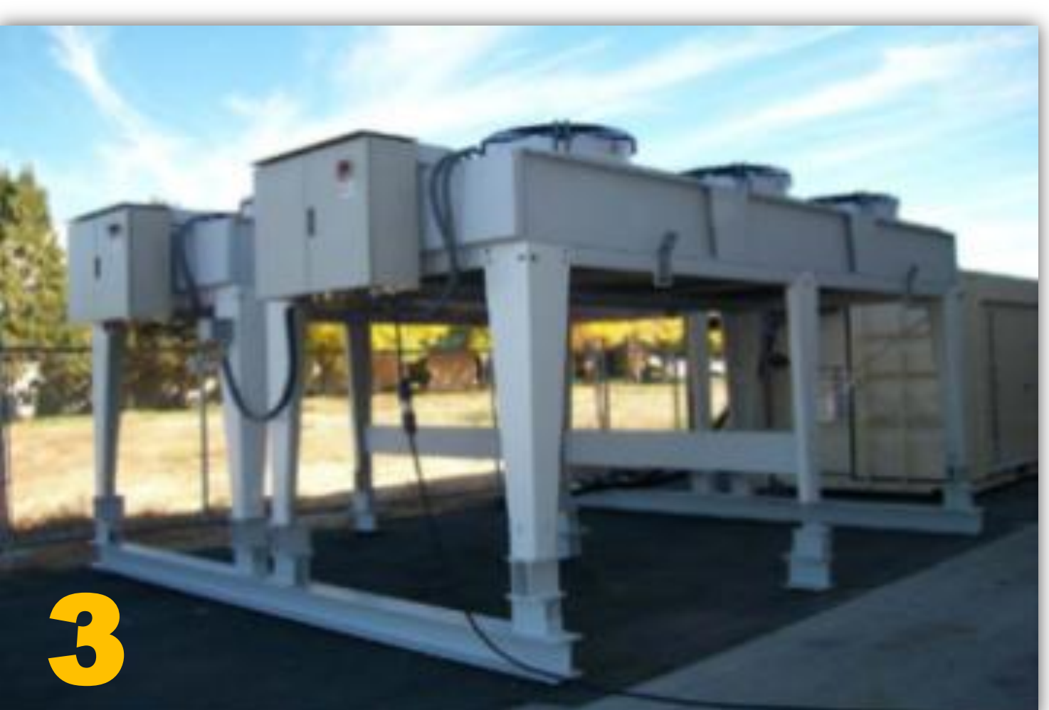
Small Scale Power Generation from Co-Produced Geothermal Fluid – Electratherm has successfully demonstrated the technical and economic feasibility of geothermal energy production through a state-of-the-art Organic Rankine Cycle (ORC) heat-to-power generator.
