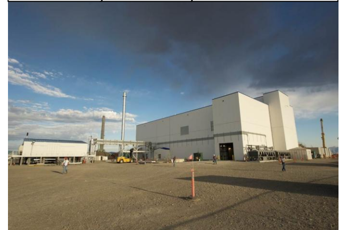
Integrated Waste Treatment Unit Facility
