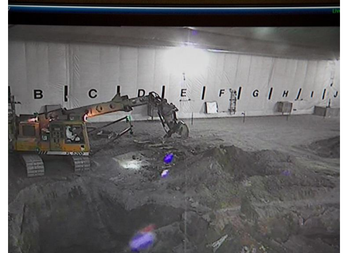
Targeted Waste Exhumations at Accelerated Retrieval Project VIII facility
