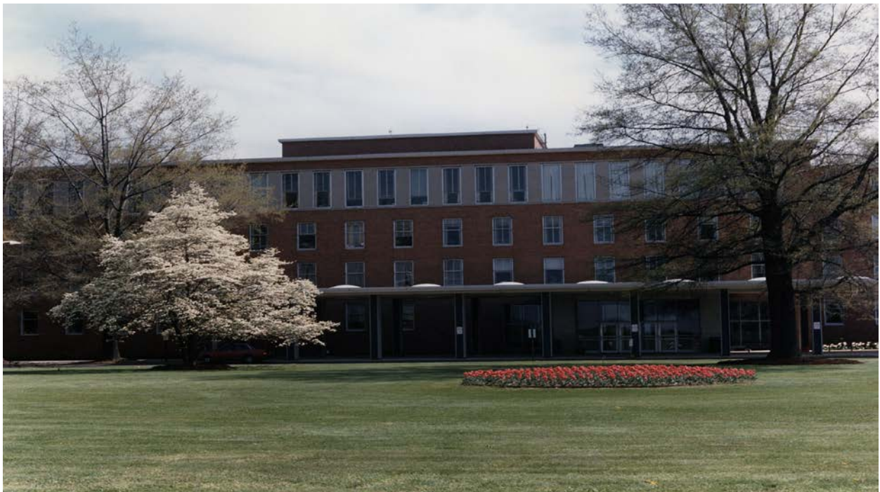
Figure 1: The DOE Germantown Headquarters Facility
