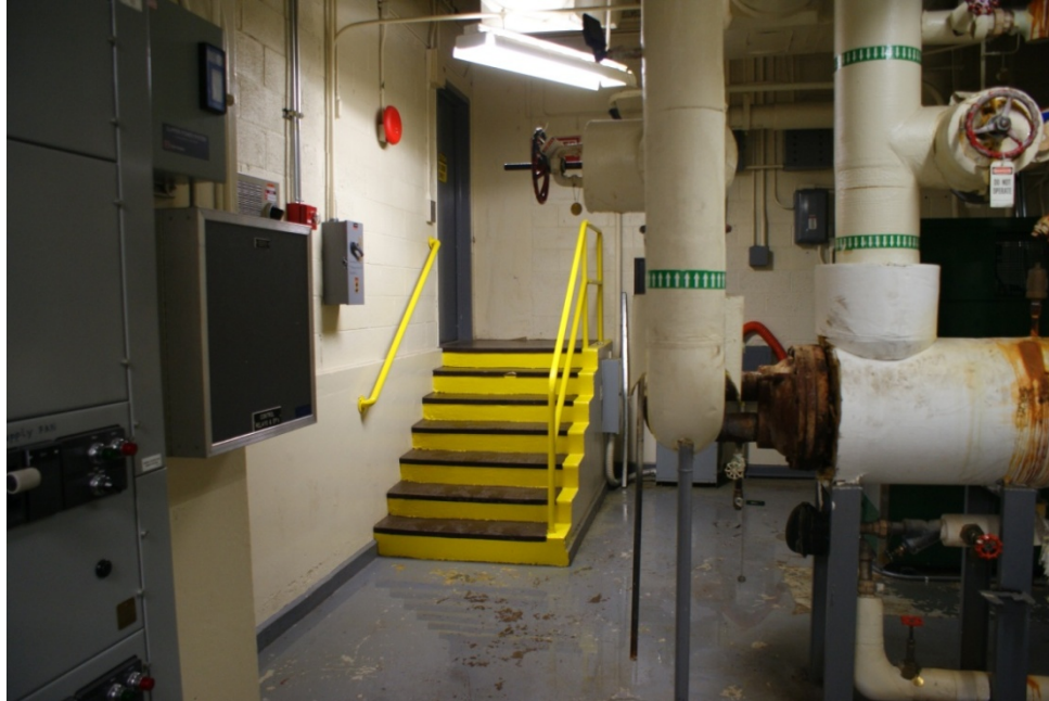
Figure 3: Mechanical Equipment Room 7 Entrance Stairs
