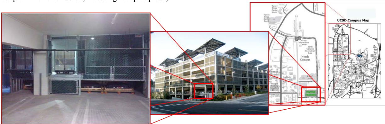
Figure III - 1: 2 nd Use Battery Field Test Installation at University of California, San Diego.
