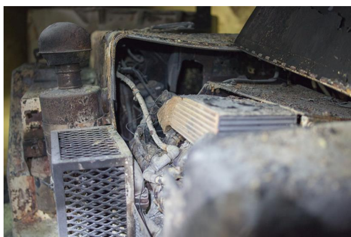
Figure 19: Engine Cooling Coils
