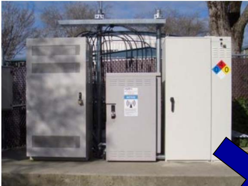
Standard Telecom Installation
