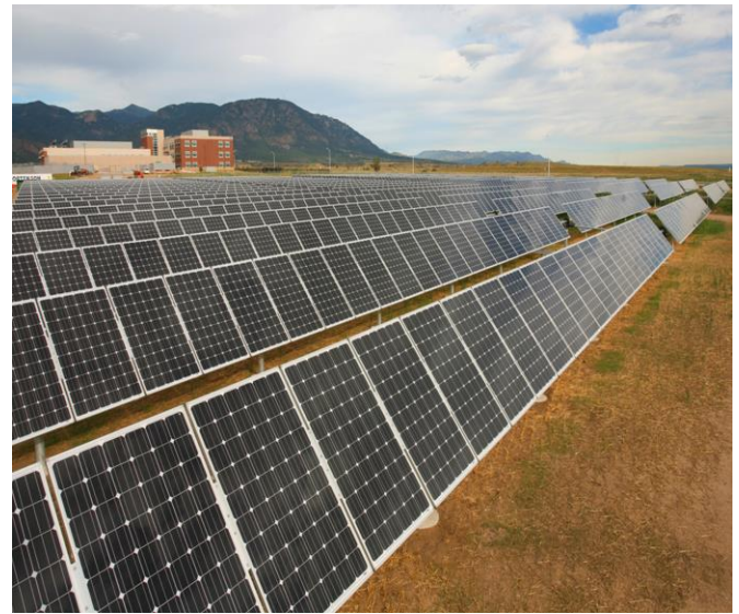
Fort Carson's first U.S. Green Building Council platinum-level Leadership in Energy and Environmental Design certified facility, the 4th Armored Brigade Combat Team Brigade and Battalion Headquarters, which features a 482-kilowatt ground-mounted, tracking photovoltaic system.
