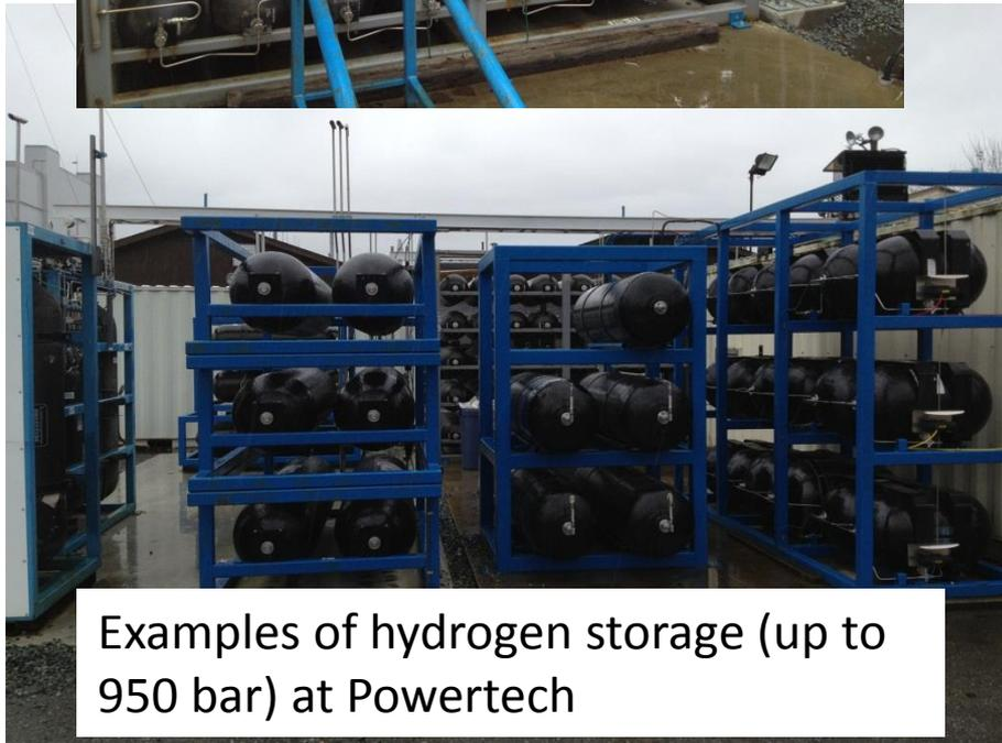
Examples of hydrogen storage (up to 950 bar) at Powertech
